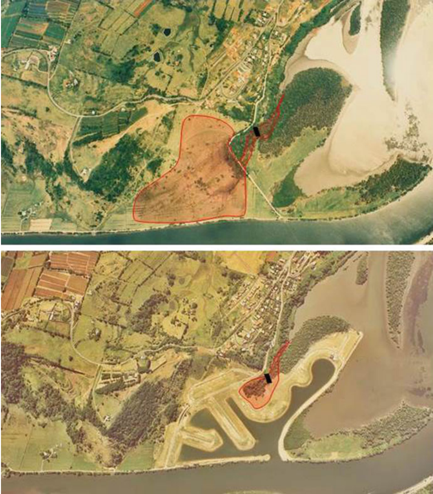
Fig. 33.4 Aerial photos from 1970s (top) and 1980s (bottom) showing the levee and catchment change that have contributed to the odour, poor water quality, weed incursion and mosquito hazard experienced by today’s residents
