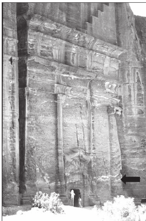
Figure 5. Weathering damage on the facade of the temples of Petra; the arrow indicates the capillary rise to above human height, illustrating the possibility of deterioration from soluble salts. Photograph: Heather Viles.
