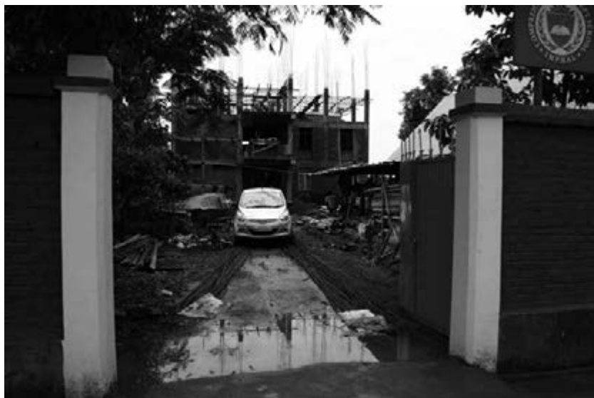
Image 7.1 School under construction, Sangaiprou
