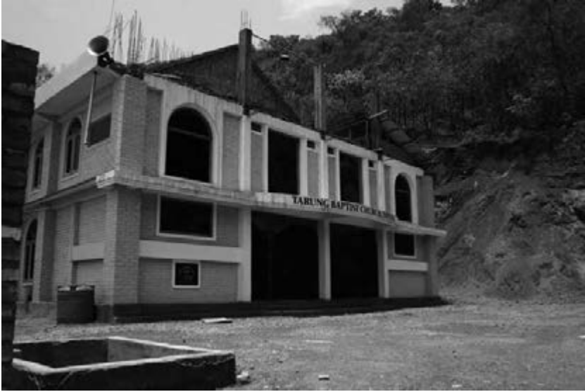
Image 6.2 Baptist church under construction, Langol
