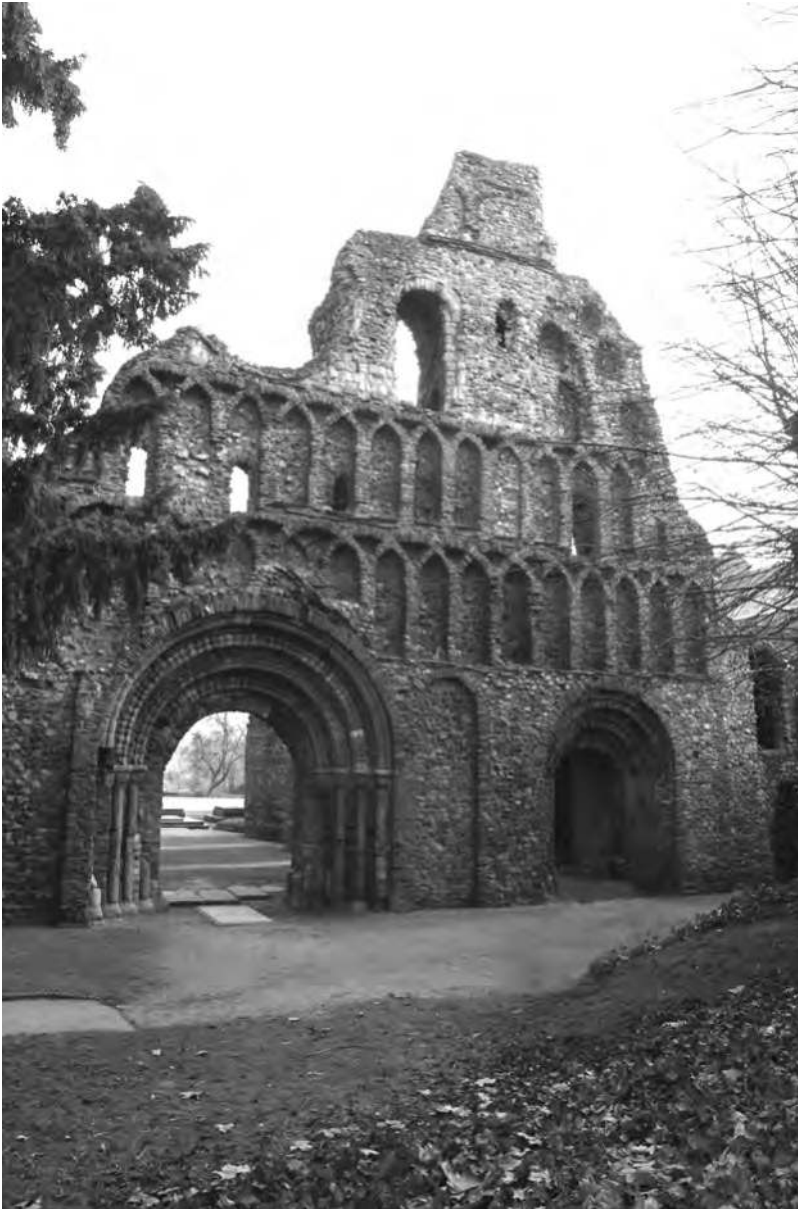
Fig 10.5 The west front of St Botolph's Priory contains the traces of the earliest major round window in England, c 1150 (Tony Nichols).
