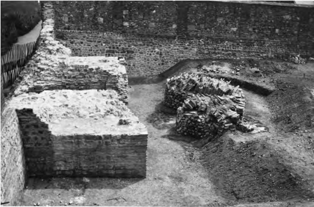
Fig 7.5 A view of Duncan's Gate taken in 1929, following its conservation, which clearly shows the separate block of fallen masonry representing part of the tower (Colchester Museums).
