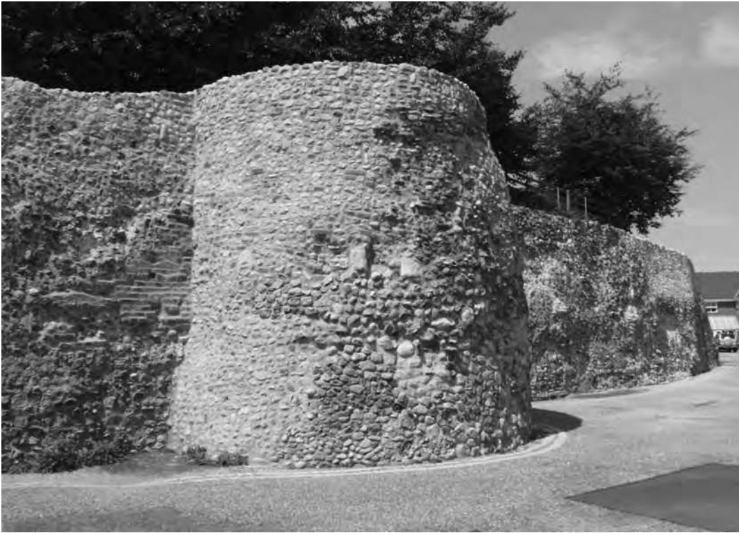
Fig 11.3 Bastion 2 in Priory Street is one of a series of external towers added to the town wall to strengthen its south-eastern corner (Philip J Wise).
