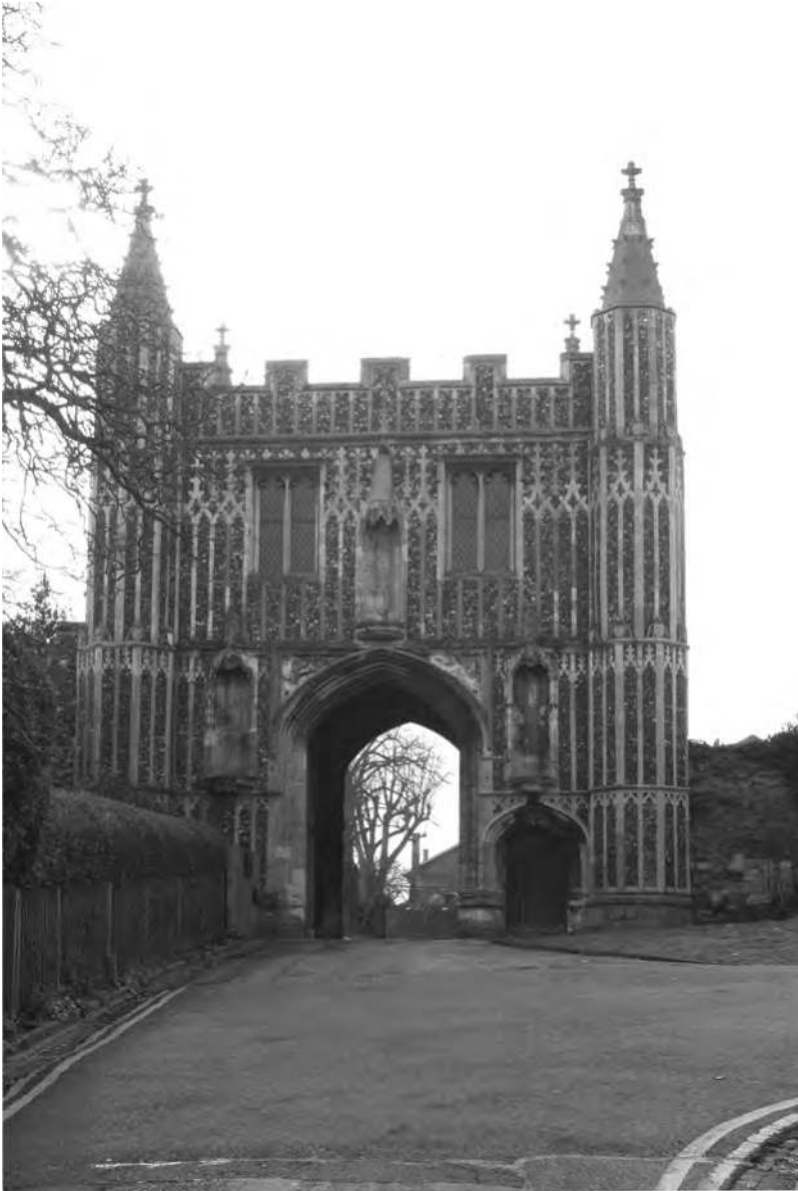
Fig 11.7 St John's Abbey gatehouse was built as a tangible expression of the power and prestige of the abbey during the 15th century (Tony Nichols).
