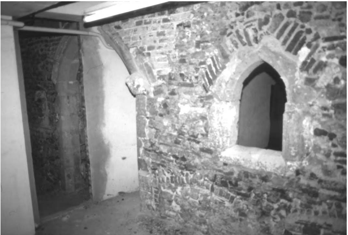
Fig 10.9 The cellar beneath 35–37 High Street showing a rubble wall with surviving 14th-century features (Philip J. Wise).
