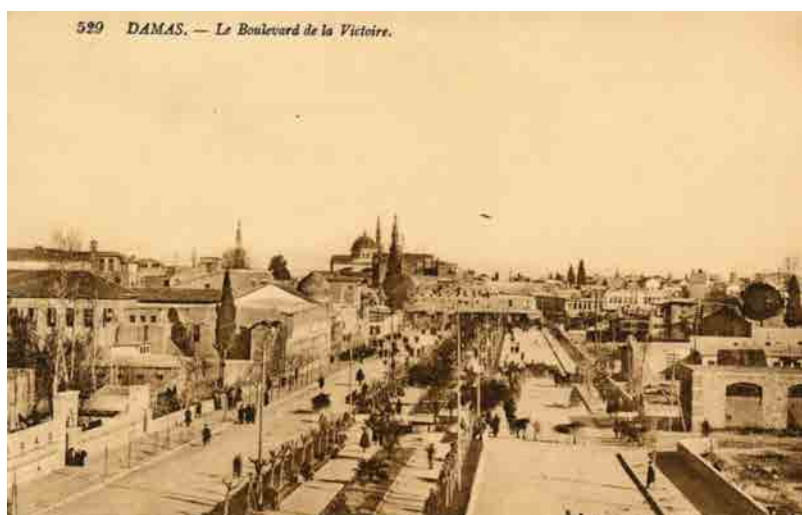
FIGURE 9.29 The middle part of Cemal Pasha Boulevard with empty plots of land (to the right of the street) (from a postcard in the collection of the author).
