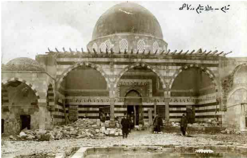
FIGURE 9.6 The Madrasa al-Salimiyya during the renovation: Damascus – The dervish lodge of Sultan Selim (Şâm – Sulţân Selîm dergâhı). Courtesy of Wolf-Dieter Lemke, Berlin.
