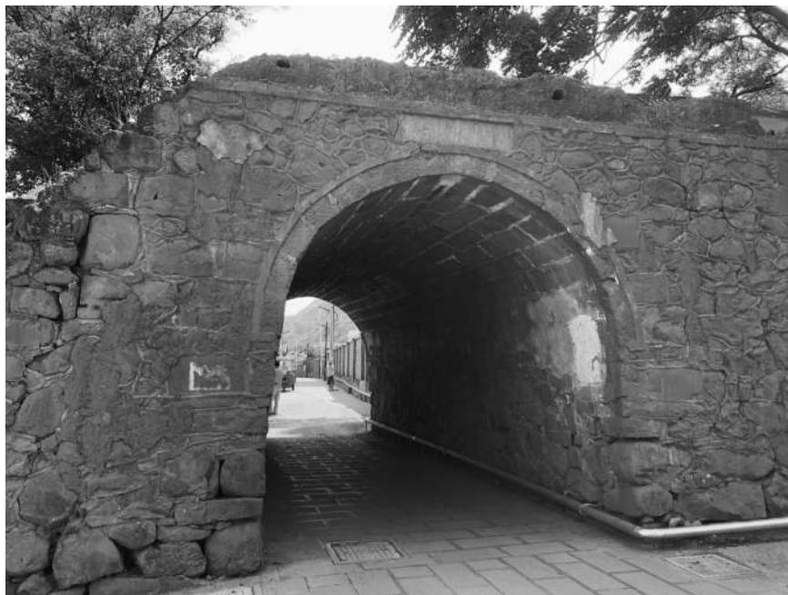
Figure 3.1 The South Gate of the Qingshui postal relay station.
