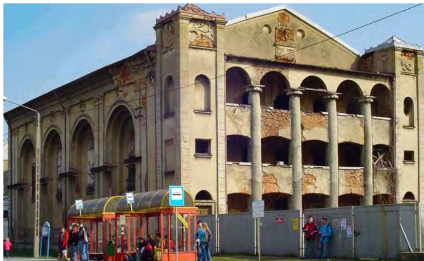
Figure 6.1. The synagogue in Dąbrowa Tarnowska, 2007. The synagogue was renovated in 2012 thanks to a seven million euro grant from the EU. It functions today as a historical museum and cultural center. Photo by Anna Hudyka. Courtesy of the photographer.
