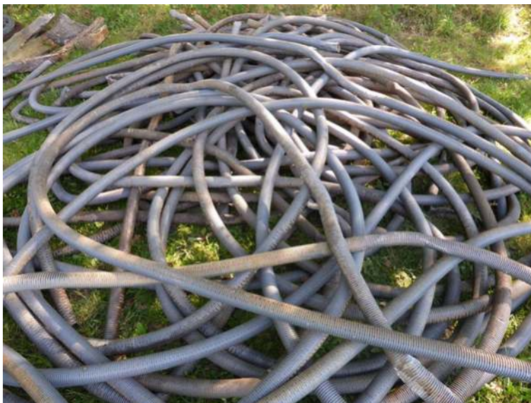
Fig. 9.4 Removed drain tubes
