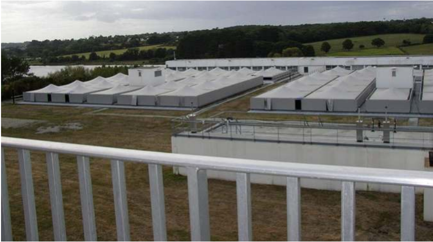
Fig. 11.1 The Drézet drinking water plant, in the Vilaine catchment. Photo Carina Furusho, 16/09/2013
