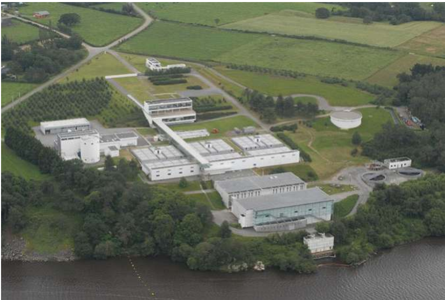
Fig. 6.4 The drinking water production plant (Drezet at Férel) that treats the water from the Arzal reservoir ( Source IAV, with authorization )
