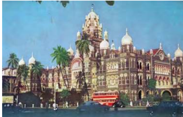
Fig. 35: Mumbai, Western Railway Office.
