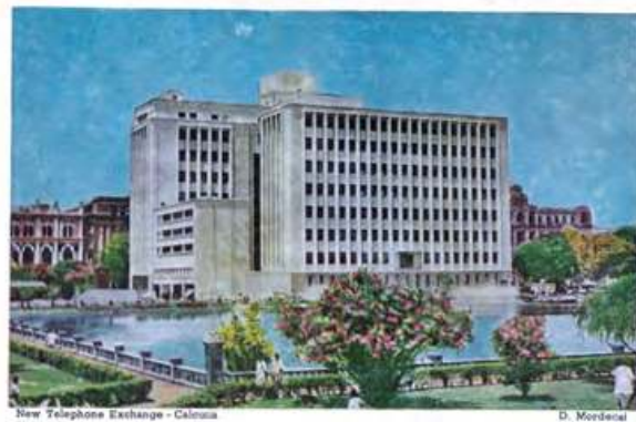
Fig. 34: Kolkata, New Telephone Exchange.
