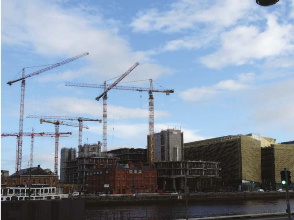
FIGURE 8.2: Construction of the Dublin Docklands. Photo by authors, 2019.
