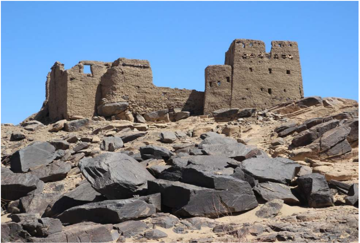
Plate 6.1. Kulubnarti, site 21-S-2. View of the 'Castle-house' from the south, taken 2014 (photo courtesy N. Spencer).
