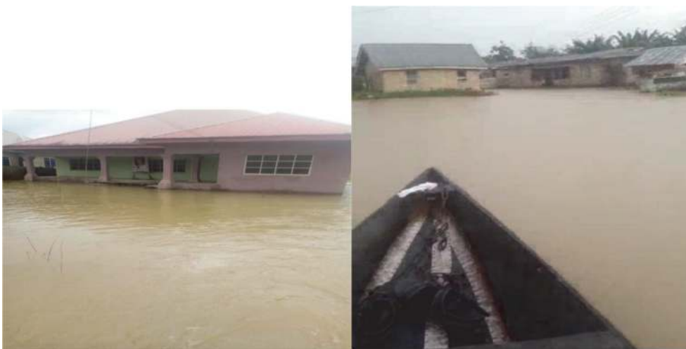
Figure 8. Flooded streets and abandoned houses where residents have migrated.
