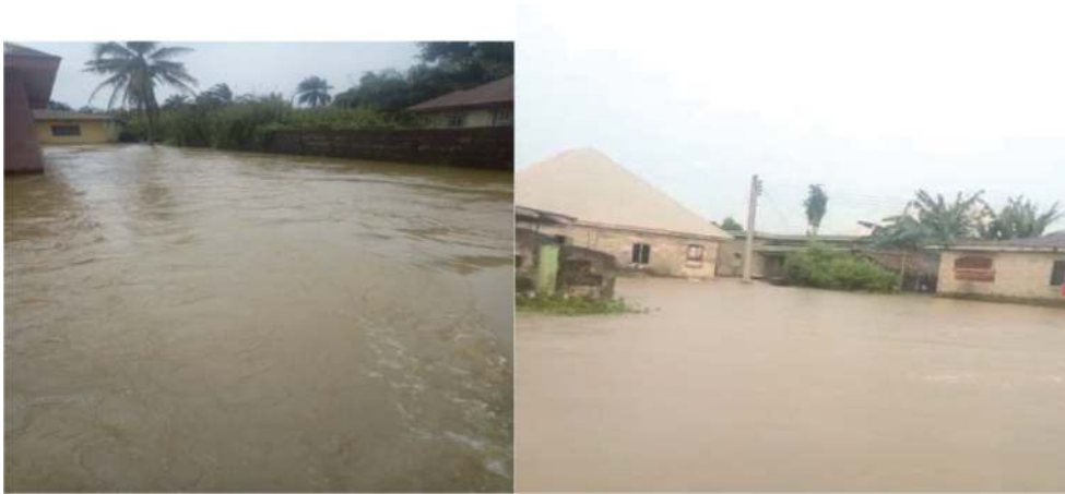
Figure 9. More flooded houses and streets that have become uninhabitable and temporarily abandoned.
