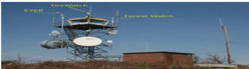
Figure 11. Tower in Tumut, Australia, with the three systems [20].
