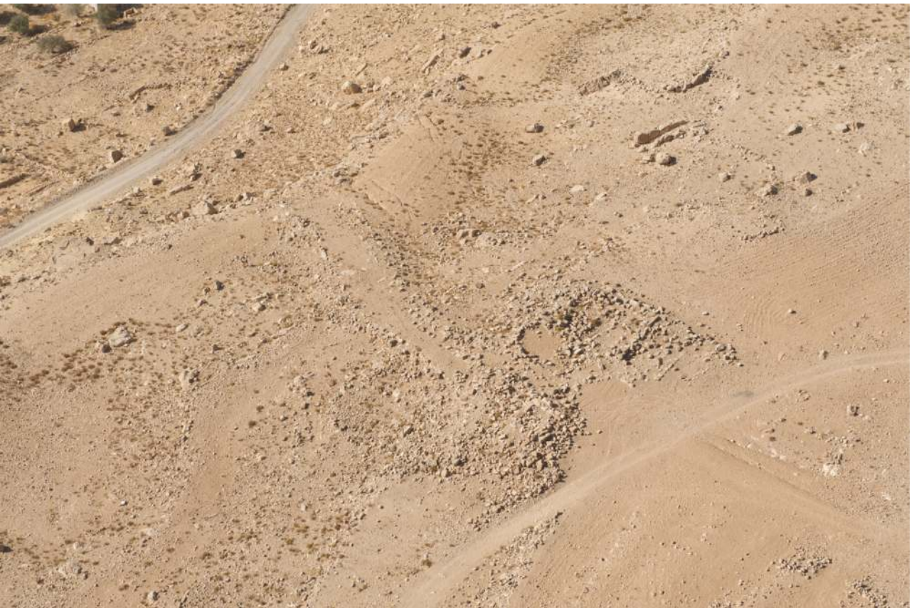
FIG. 276 Aerial view of the possible fortlet/road station of Khirbet ar-Rakham. Photo: APAAME.
