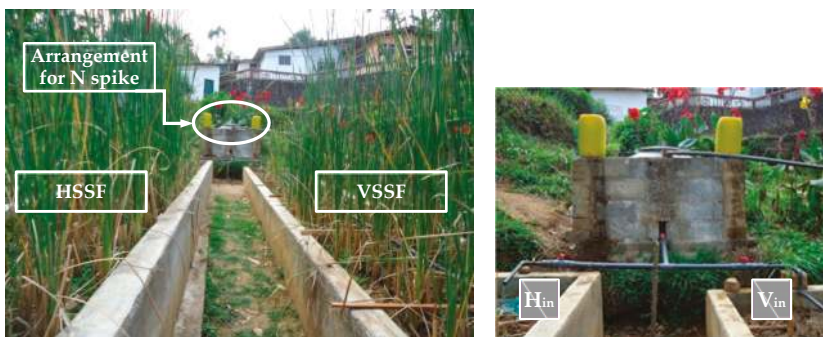
Figure 6. Arrangement for nitrogen (N) supplementation to the wetland units, H_{in} : Influent to the HSSF unit and V_{in} : Influent to the VSSF unit.
