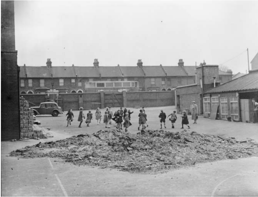
Figure 4.3 Children playing next to a bomb crater full of rubble in the playground of Lombard Wall School, South East London. © Imperial War Museum, D 3170.
