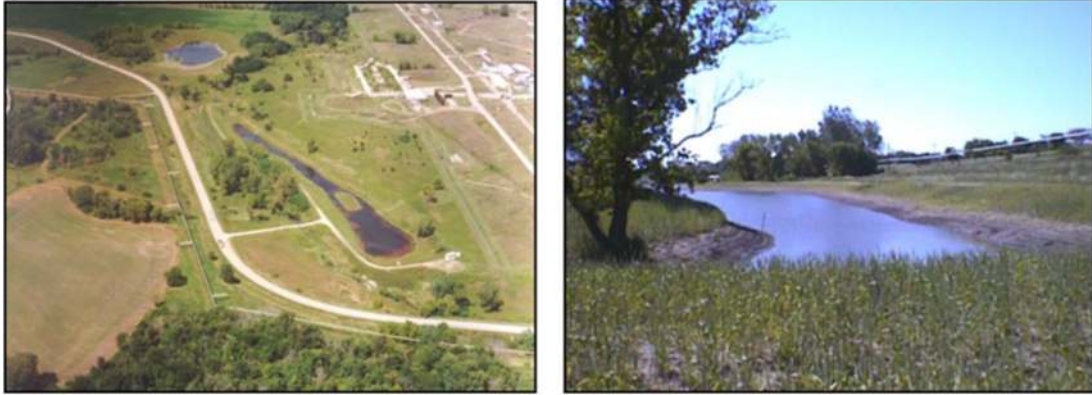
Figure 12.4 Aerial view (left) and photo of the inlet to the horizontal flow, free surface pond at the Iowa Army Ammunition Plant in Middletown, Iowa. It is planted with arrowhead (native vegetation) and resulted in the treatment of RDX contaminant to meet required effluent discharge permit.
