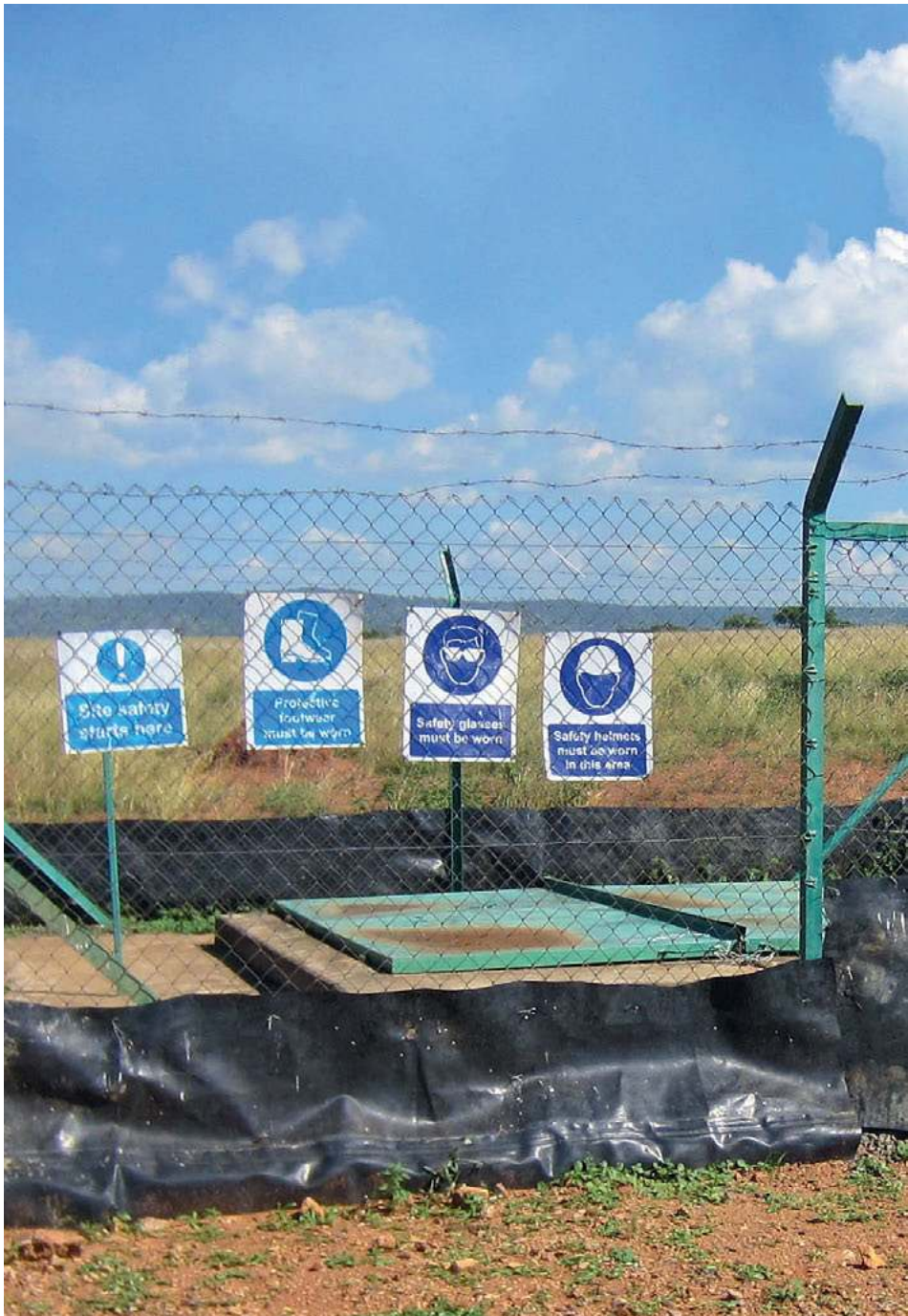
Figure 19: Closed well with safety warnings, Hoima district (2012).
