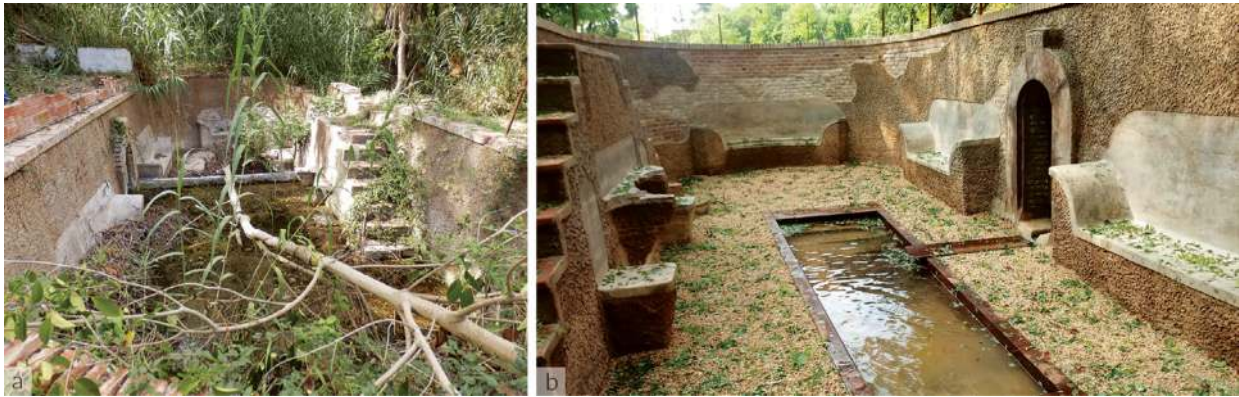
Figure 3.6a and b The Can Moritz spring, Rubí, a) before and b) after the final renovation (Source: Mireia Gascon)
