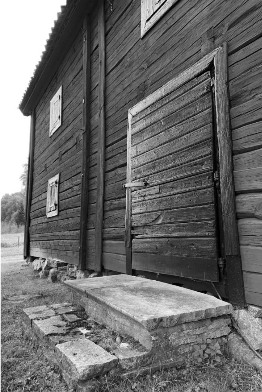
FIGURE 11.3 Fragments exposing and imposing deception. An elaborate stone slab used as a threshold for the “Mustering Barn”. It is most likely reused from a previous building, possibly the torn-down wing attributed to the King’s visit (photo: Anna Röst).
