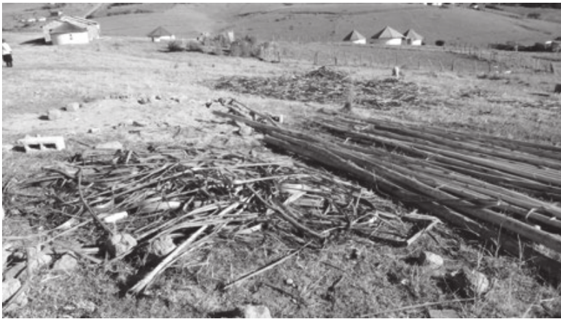
FIGURE 13.5: Wood from the local forest being stripped for use as rafters for the roofs of the rondavels, illustrating indigenous ways of building.
