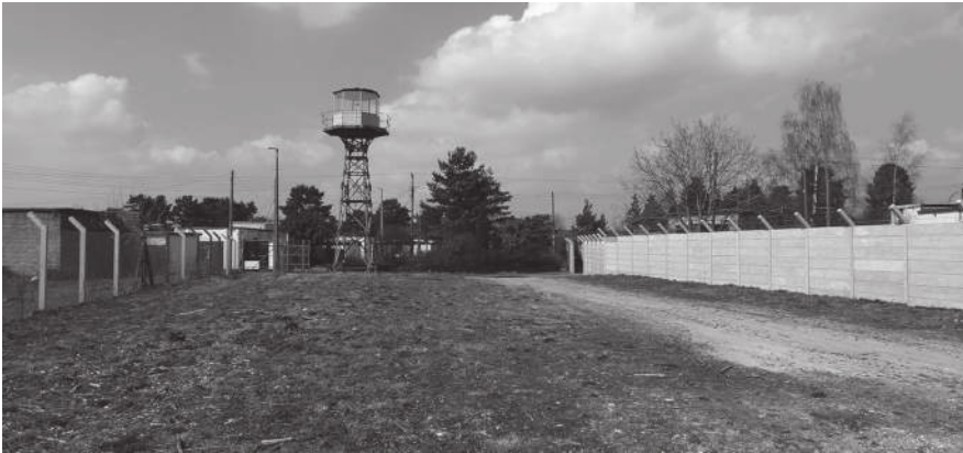
Fig. 2: Barnham, Suffolk, early 1950s atomic bomb store, conservation on this scheduled monument has included the conservation of its watchtowers and the replacement of sections of its outer fences. © W D Cocroft
