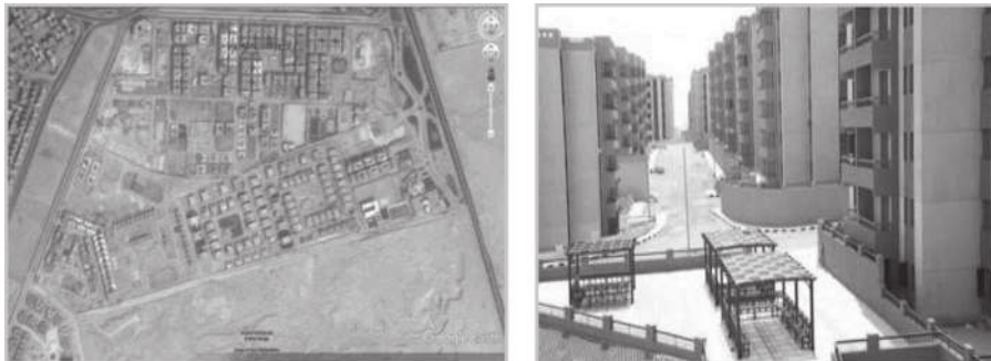
Figure 7. Buildings and streets in the Asmarat district project.
