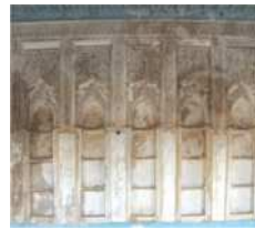
Figure 43. Wall slots inside the Hussein Rifai house.
