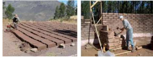
Figure 16. Left and right, illustrate adobe blocks & architecture. (claysandstraw, 2005), (d2wpnc0srowh1f.cloudfront.net, 2014).
