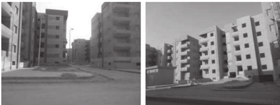
Figure 8. Buildings and streets in Imbaba Airport.
