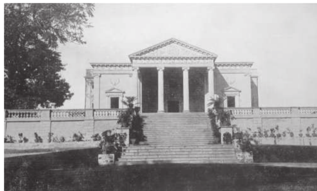
Figure 3(b). The Bashirbagh guest house after intervention.
