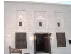
Figure 28. Façade of the Ahmed Munawar Al Rifa'i house (AD 1922).
