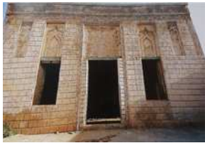
Figure 37. Details of the main portal of the Hussein Rifai house.
