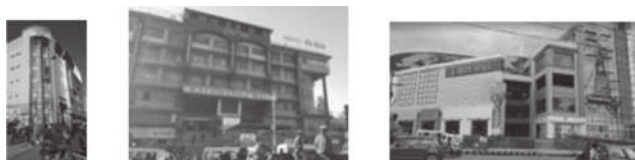
Figure 6. New commercial built forms in the major commercial hub of Kathmandu (Sources: (left, middle) Site visits; (right) Retrieved from www.labimmall.blogspot.com ).
