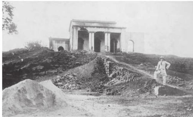
Figure 3(a). The Bashirbagh guest house before intervention.
