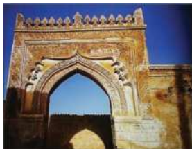
Figure 33. Front façade of the Ahmed Munawar Rifai house, with sunk or recessed arch, overlooking the street (14th century AH/20th century AD).
