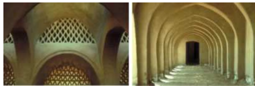
Figure 2. Architect Hassan Fathy used mud brick as a local construction material in the project New Baris Village, Kharga, Egypt. His design represents an ideal expression for the architectural identity for this particular location. (Archnet, 2014).
