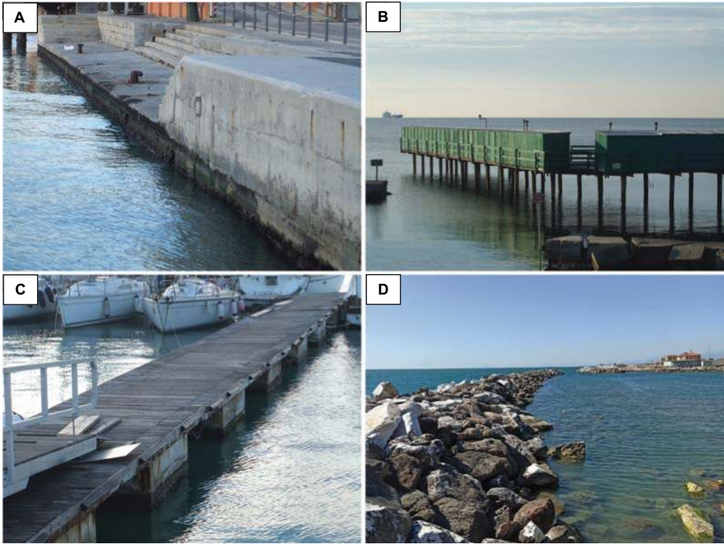
Figure 1 Examples of common coastal artificial structures: (A) seawall; (B) pier pilings; (C) floating pontoons; (D) breakwater. [Photo credits: Fabio Bulleri (A-C) and Michele Magri (D).]
