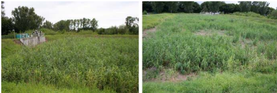
Figure 6.1 Case study 1 – CSO treatment wetland (Germany).
