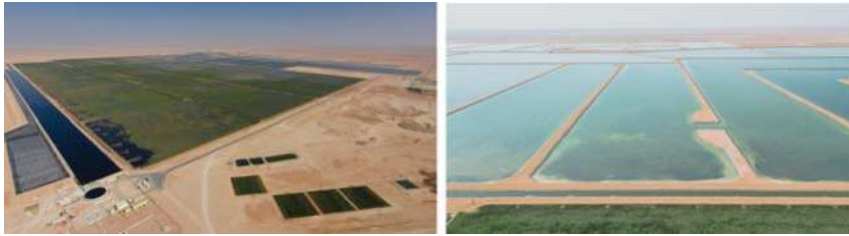
Figure 6.5 Case study 4 – Nimir Water Treatment Plant (Oman). (Pictures reprinted with permission from Bauer Nimir LLC)
