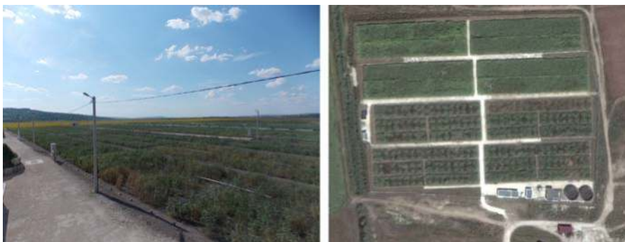
Figure 6.9 Case study 7 – Orhei Wastewater Treatment Plant (Moldova).
