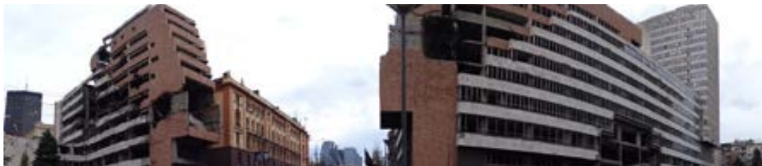
Figure 2.58. Panoramic view of the damage caused to Dobrović's Federal Ministry of Defense buildings by NATO bombing. These were the strongest signature of socialist urbanism in the tissue of old Belgrade. Left standing as a reminder of the bombing, they were finally demolished in 2015. Photo credit: Adam Jones (Creative Commons Attribution-Share Alike 2.0 Generic license - https://commons.wikimedia.org/wiki/File:Panorama_of_Buildings_Damaged_in_1999_Kosovo_War_-_Belgrade_-_Serbia_(15803615912).jpg )
