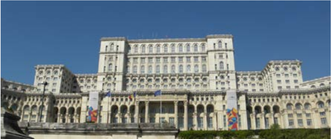
Figure 2.140. Ceaușescu's People's Palace in Bucharest: the biggest building in Europe and second-biggest in the world. This is only the apex of the project which included the long Victory of Socialism Boulevard with large multifunction buildings, coordinated in design, lining both sides of the street. Photo credit: Vi Ko (CC BY-SA 4.0).
