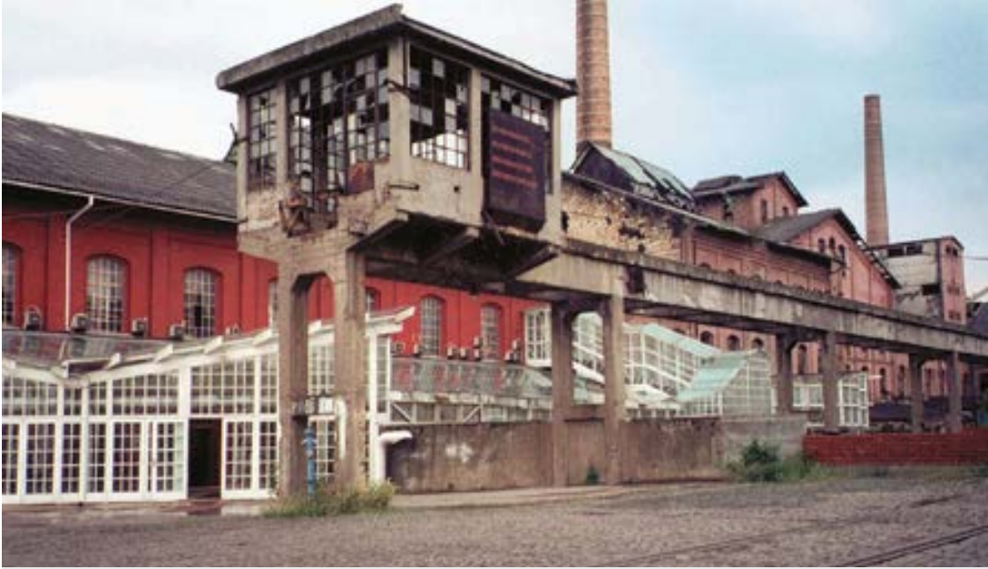
Figure 2.144. An opera house in an (industrial) desert: this abandoned sugar refinery was transformed into the "International Art Center Šećerana." Note the new glass additions which contrast with the old broken windows above ground level. Photo credit: author.
