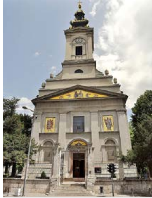
Figure 2.35. The Tower of St. Michael's Orthodox Cathedral is a significant vertical in Belgrade. Photo by Dragoljub Zamurović (Creative Commons license 3.0).
