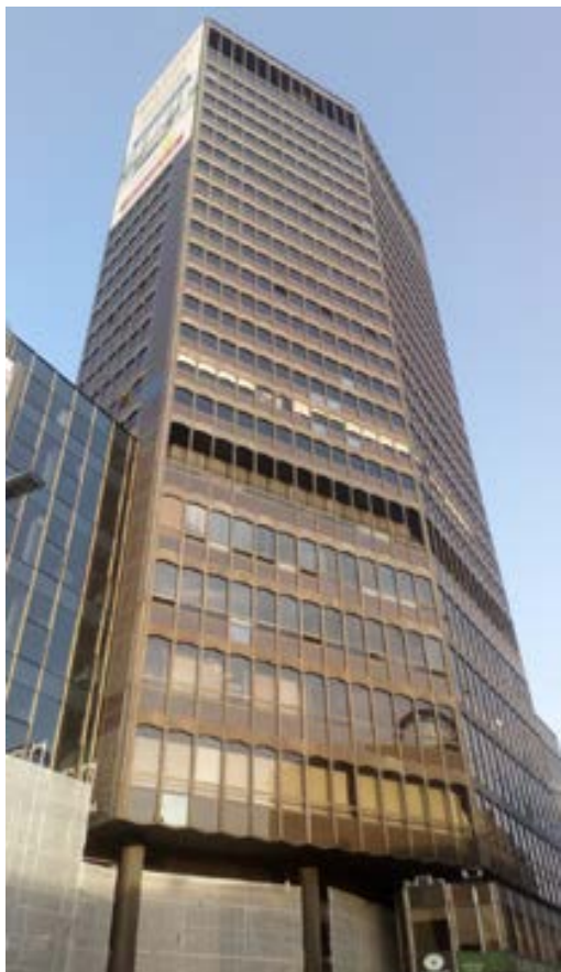
Figure 2.48. The Belgrade Palace (colloquially known as Beogradjanka), designed by Branko Pešić, the architect who also completed the design of the Temple of Saint Sava in Serbo-Byzantine revival style. Photo credit: https://forum.beobuild.rs/threads/palata-beograd-beogra%C4%91anka.4714/page-11#post-881103
