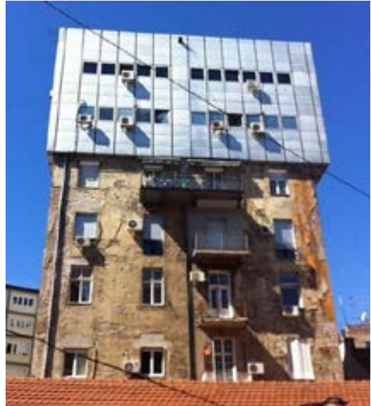
Figure 2.54. Extra floors added to a building in Belgrade. Photo credit: Instagram/malo_smo_nadogradili
