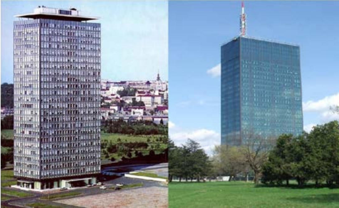
Figure 2.61. Left: the “CK” building (headquarters of the League of Communists) before being damaged by NATO missiles in 1999 (photographer unknown). Right: the same building, repaired and renovated as the “Ušće Business Center” (photo by Jelena Irić).
