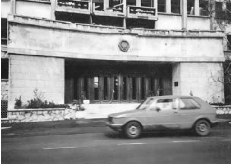
Figure 2.62. The Federal Secretariat of Internal Affairs on Kneza Miloša Street is one of the rare “socialist realist” buildings in Belgrade. An urban legend says it was built with stones from Tito’s prison camp for his ideological opponents. Photo credit: author.
