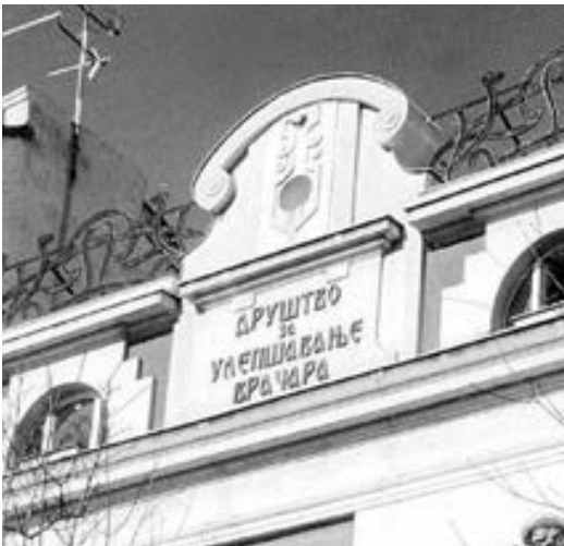
Figure 2.105. Building of the Society for the Embellishment of Vračar on Njegoševa Street. The “Miroslav” typeface is more convincing on older buildings. Photo credit: author.
