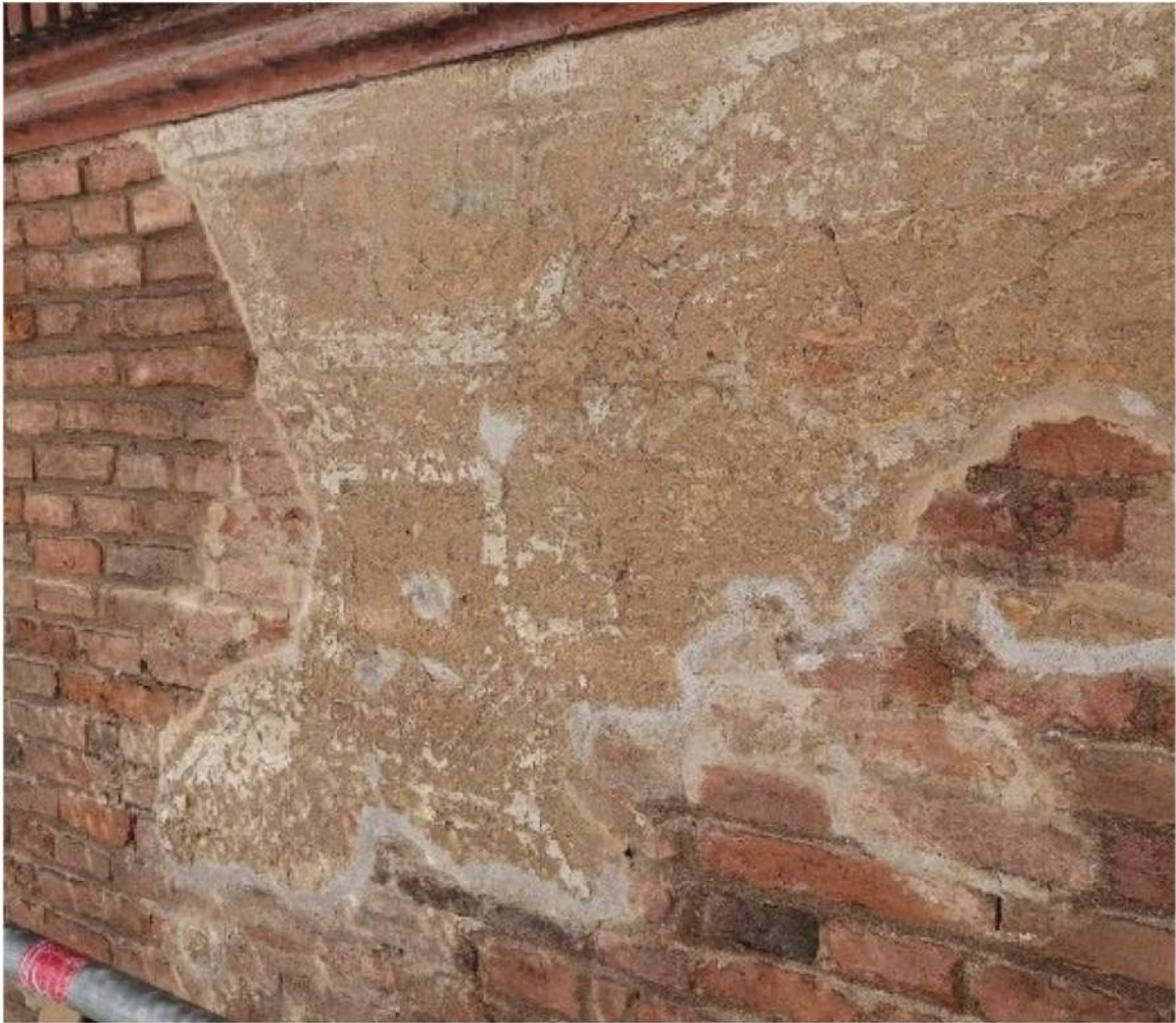
Figure 21. Restoration of plaster fragments.
