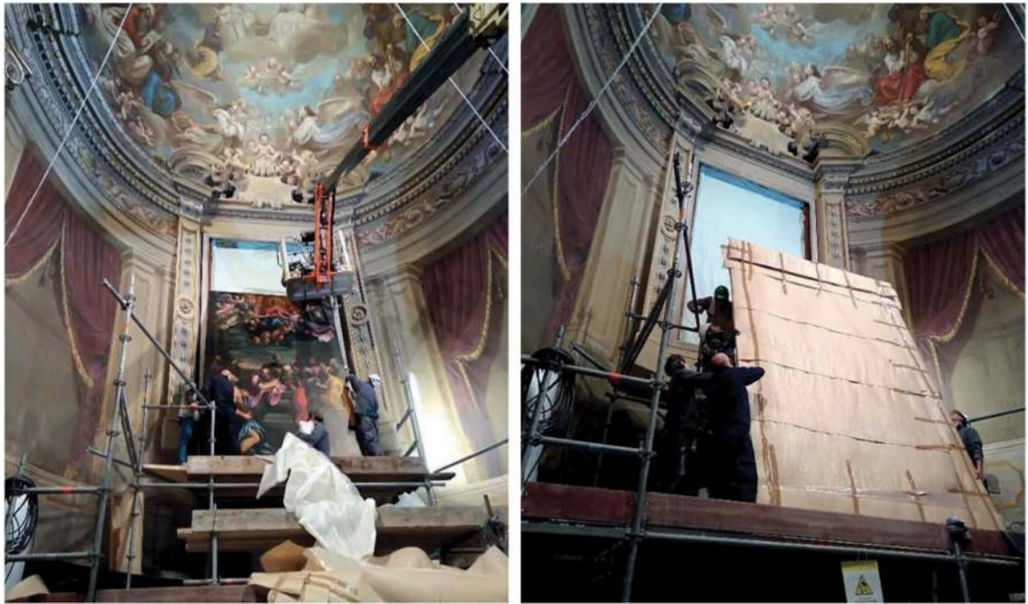
Figures 19-20. Securing operations by the fire brigade with the supervision of a MiC official personnel.
