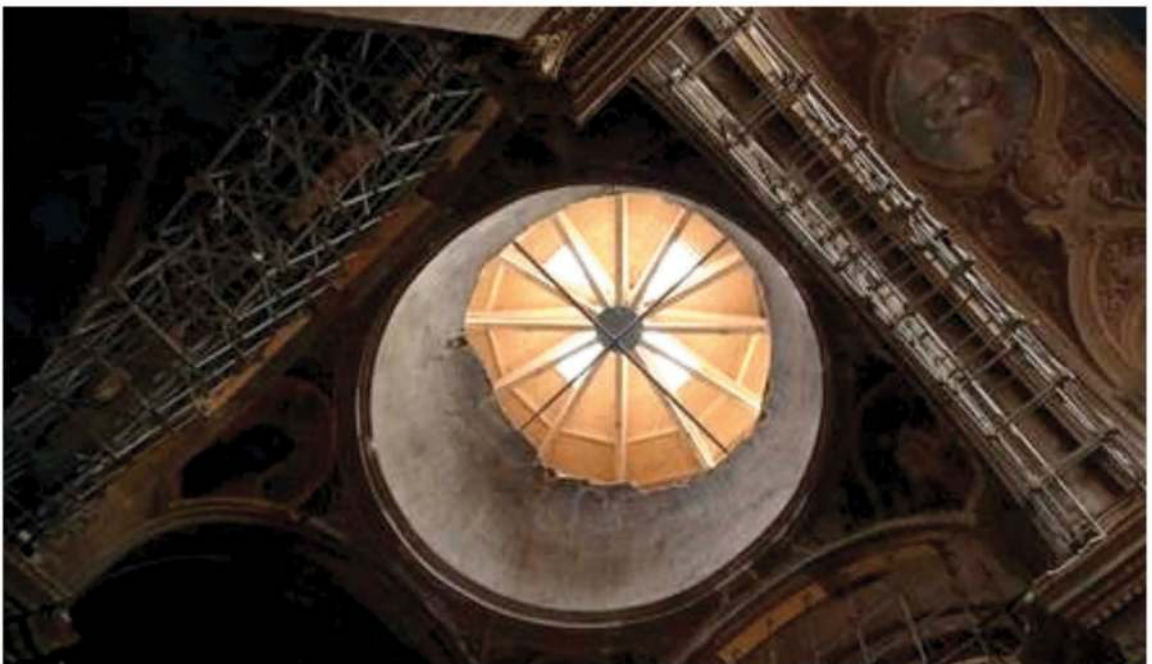
Figures 1-2. Picture of the dome seen from below before and after the temporary cover had been put in place.
