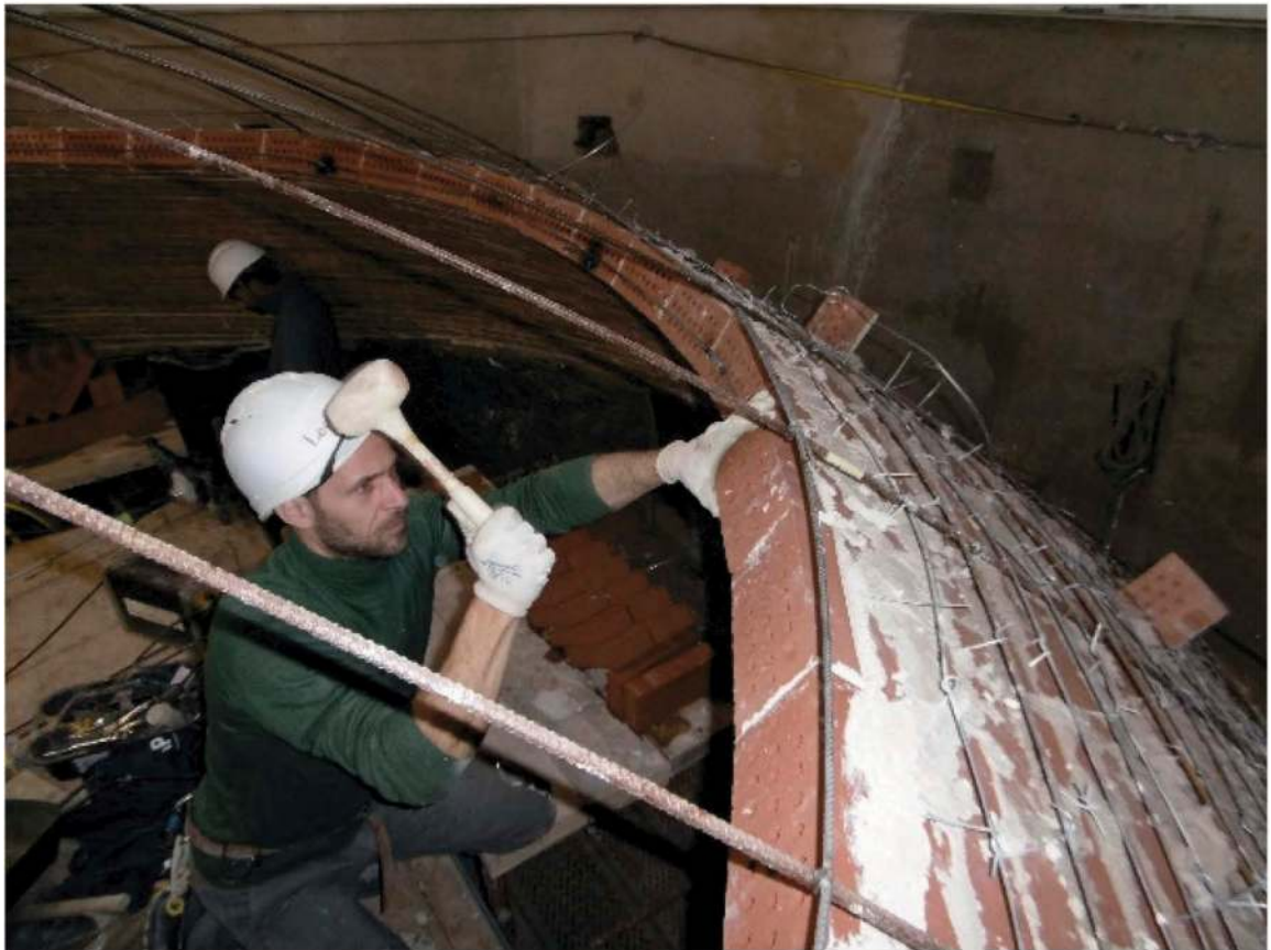
Figures 14-15. The phases and methodology of the construction: extradossal rib made of metal rods and laying of the brick elements from inside the wall cap under construction.
