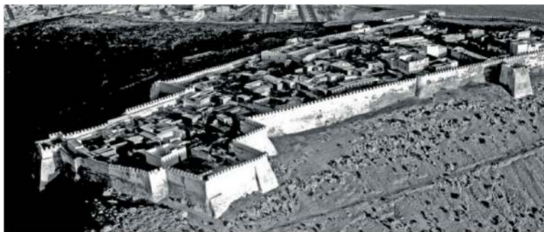
Figure 9. Agadir Oufella, The Historic Kasbah, Before the earthquake 1960.
