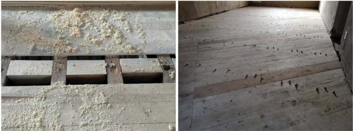
Figure 16. Insertion of wooden beam segments in the extrados between the rafters - Stiffening and consolidation of slabs by means of triple planking and connectors.
