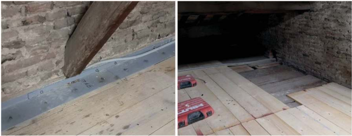
Figure 15. Stiffening of attic slabs and metal curbs.
