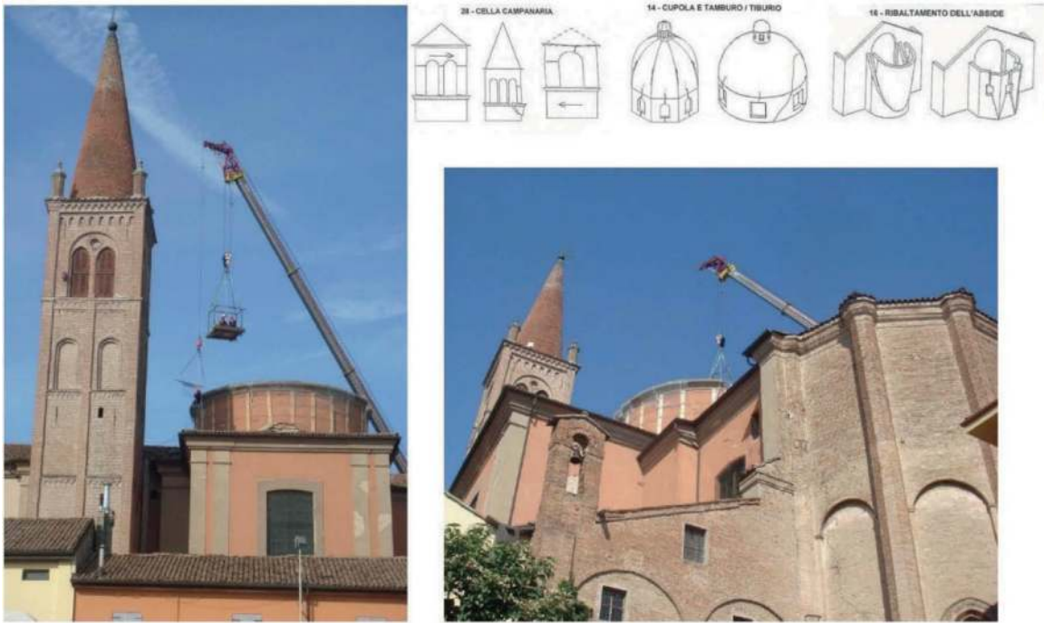
Figure 6. A few images of the damage, representative of the most prevalent damage found, with indications of the respective mechanisms as filled in the damage survey forms.
