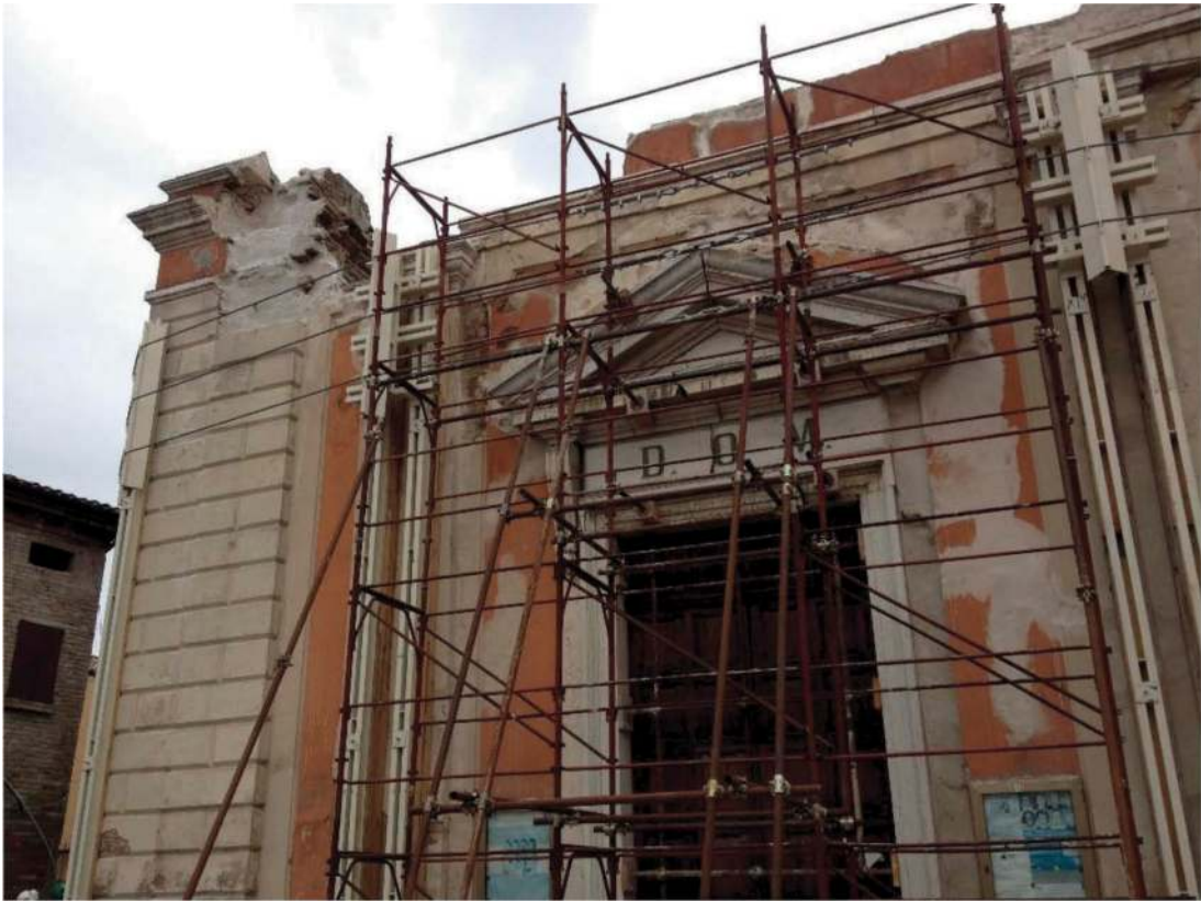
Figure 4. The first phase of securing the Church of San Felice: the scaffolding framework to prevent the overturning of the walls.
