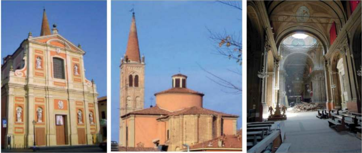
Figure 7. Images of the Collegiate before the 2012 earthquake (on the left) and an image of the collapse taken during the damage survey by the MiC official (on the right).
