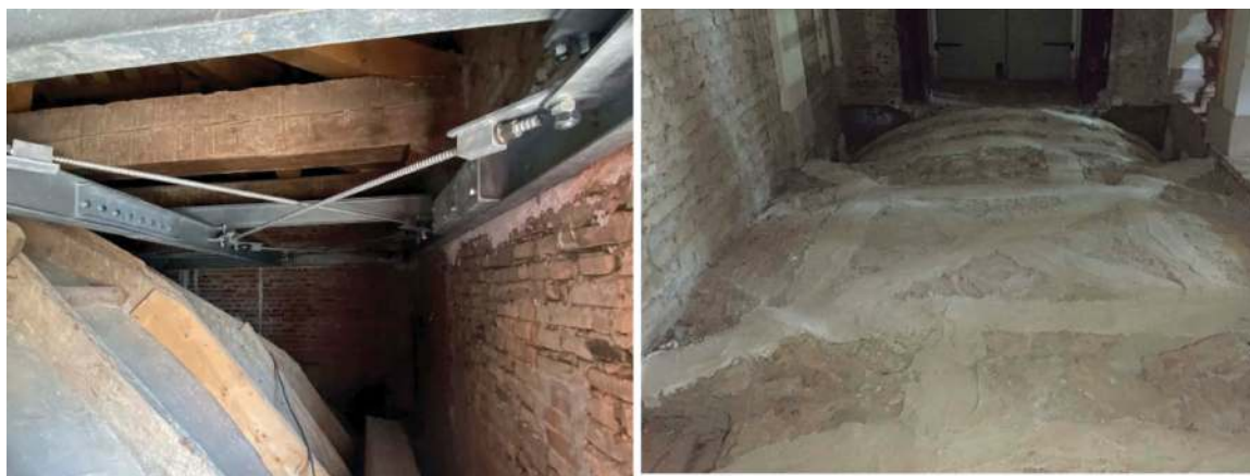
Figure 27. Images of structural reinforcements on the intrados of the vaults. A large two-dimensional steel girder lattice will make any movement of the central tower's masonry more difficult.
