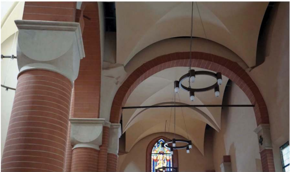
Figures 1-2. Mirandola Cathedral in its final state after restoration. Above, general view of the Central Nave; below, detail of the Left Side Nave.
