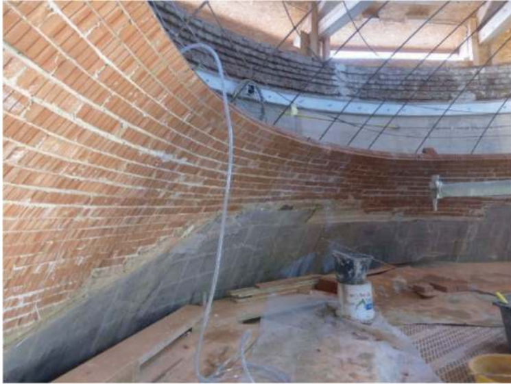
Figure 16. The internal brick elements from inside the wall cap.
