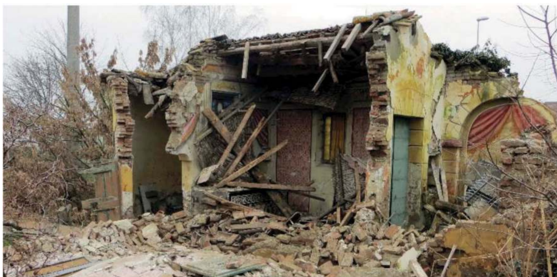
Figure 1. Mirabello, Ferrara. The Oratory of the Beata Vergine di San Luca, safety procedures and reconstruction in a single phase.
