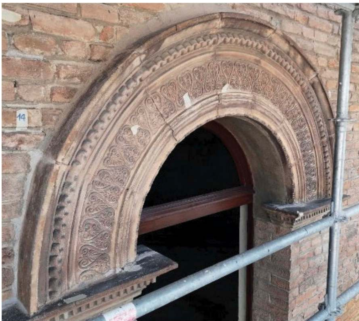
Figure 22. Restoration of plaster fragments and window surrounds.
