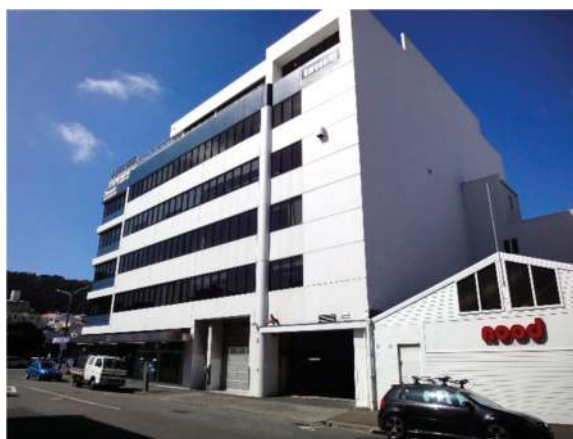
Figure 4. This large commercial building dating to the 1980s is the second least liked building in College Street.
