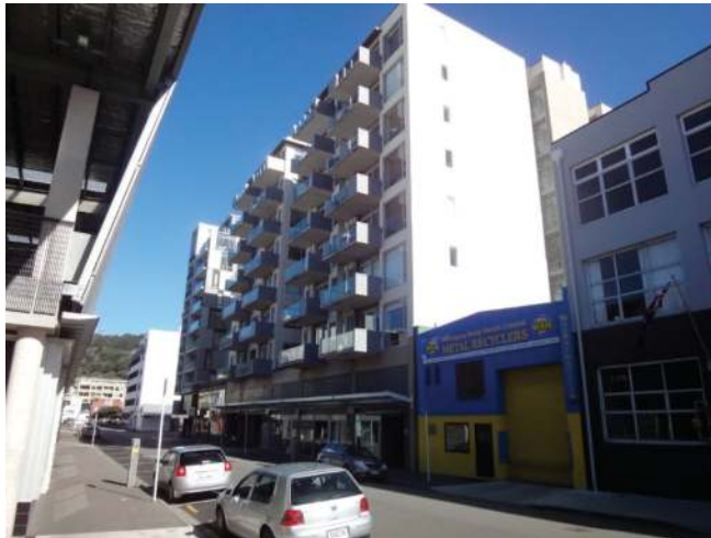
Figure 7. The Trinity Apartments building, in the middle, establishes a poorly regarded relationship with its neighbours. The public also dislike the large blank side wall and the private balconies projecting beyond the site and into the public street space.
