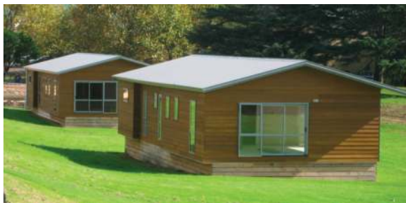
Figure 4. Control house (foreground) and test house.
