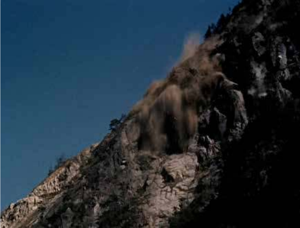
Fig. 8.4. Blasting in Sakuma Dam . Picture courtesy Documentary Film Preservation Center, Japan.
