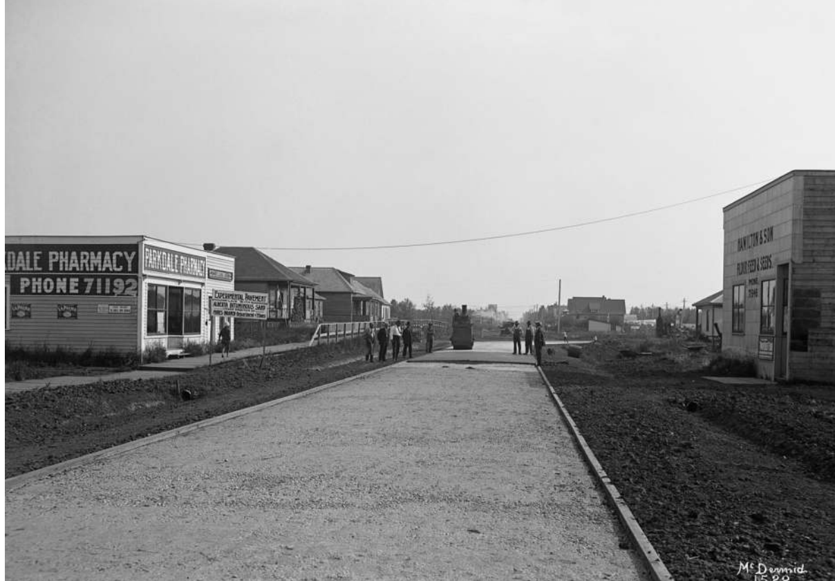
Experimental asphalt paving in Edmonton, Alberta, in 1915 using tar sands from Fort McMurray. McDermid Studio, Glenbow Archives, NC-6-1522.
