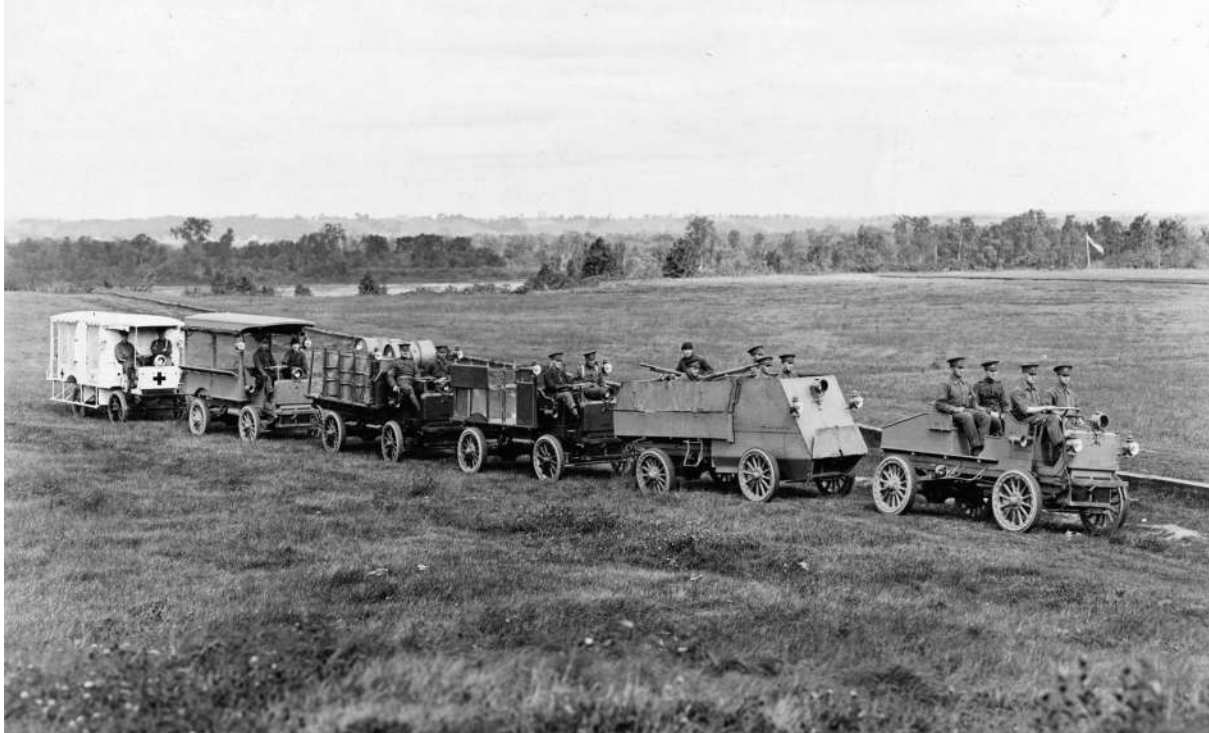
Vehicles of the Canadian Automobile Machine Gun Brigade No. 1 moving to the Rockcliffe Ranges, Ottawa, for inspection by the Governor General on 23 September 1914. All variants of the 20 trucks purchased from the Auto Car Company of Ardmore, Pennsylvania, can be seen. Right to left: officers' liaison vehicle, "Auto Car" armoured car, general transport vehicle, shop van and ambulance. Photo courtesy of the Musée Héritage Museum, St. Albert.
