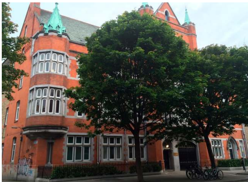
Figure 1. Street façade of Hatch Hall, Dublin, Ireland; photo taken by author.
