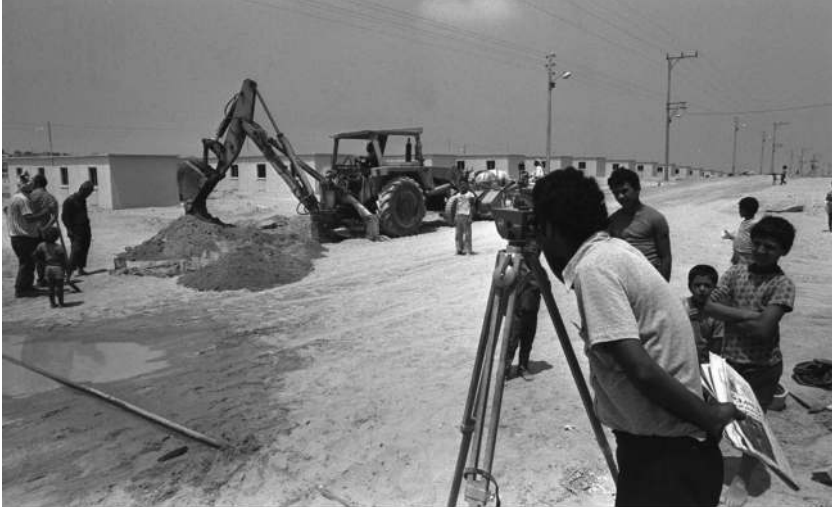
Figure 6. PWD during the construction works at Sheikh Radwan Neighbourhood, 1976 (National Photography Collection, photo by Moshe Milner).
