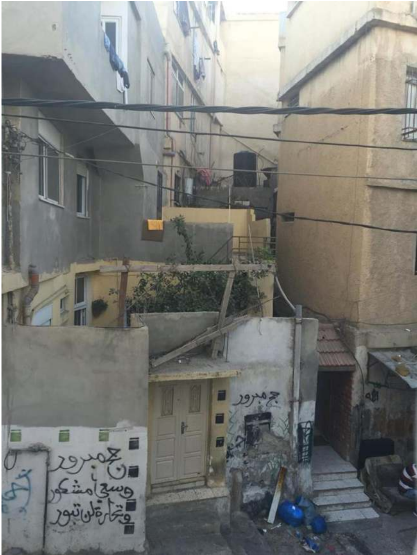
Figure 4. Incremental housing in Al-Amari. Buildings have progressively expanded, saturating the ground floor of the respective plots. Source: the author.
