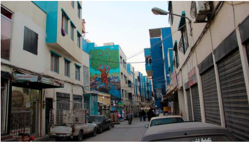
Figure 4. Rebuilt areas of Nahr Al-Barid. As of 2017, only 45 per cent of the camp's population has been able to return to the site; photo sourced from Starr (2017).
