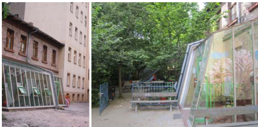
Figure 5. Heide Moldenhauer, Kita (day care centre) in Block 78, Kreuzberg, Berlin, when built in 1984, and in 2012; photographed by Heide Moldenhauer and Esra Akcan.
