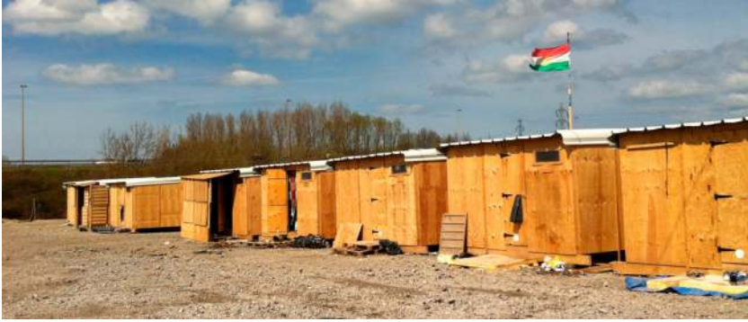
Figure 3. The prefabricated shelters in the MSF camp near Dunkirk where the reappropriation could already be seen; photo taken by author in April 2016.
