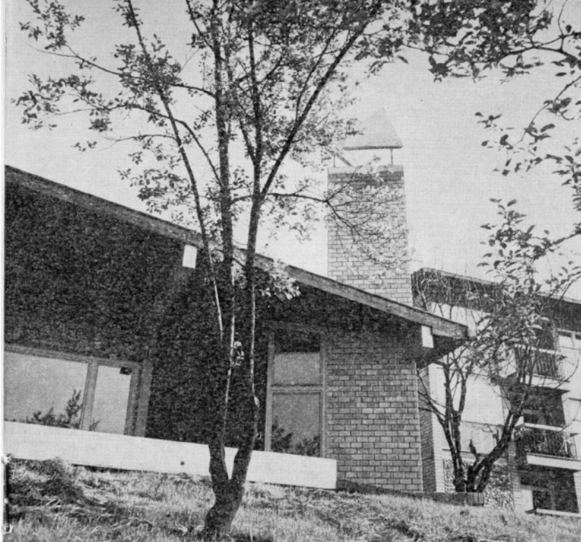
Figure 7. United Nations Refugee centre in Banja Koviljača. Architect Mihajlo Mitrović, 1964. Detail of the façade (source: Mihajlo Mitrović: izložba arhitekture, Muzej primenjene umetnosti Beograd, 13-25 April 1971 ).
