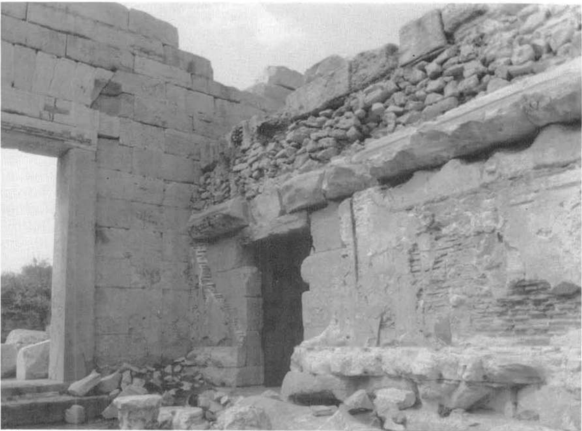
(b) Severan Temple: south side of podium, showing entrance to vaults.
