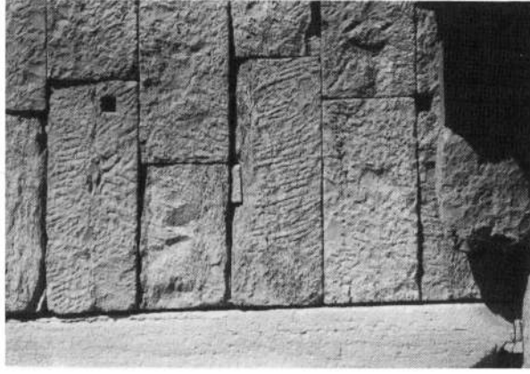
(d) Colonnaded Street: the opposite face of the wall illustrated in (c).
