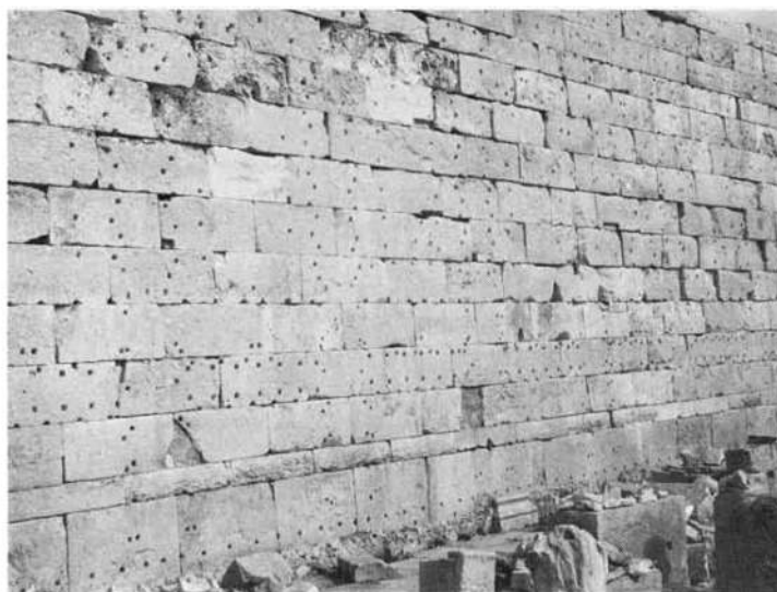
(d) Forum: fixing-holes for the veneer on the inner face of the north-west perimeter wall.
