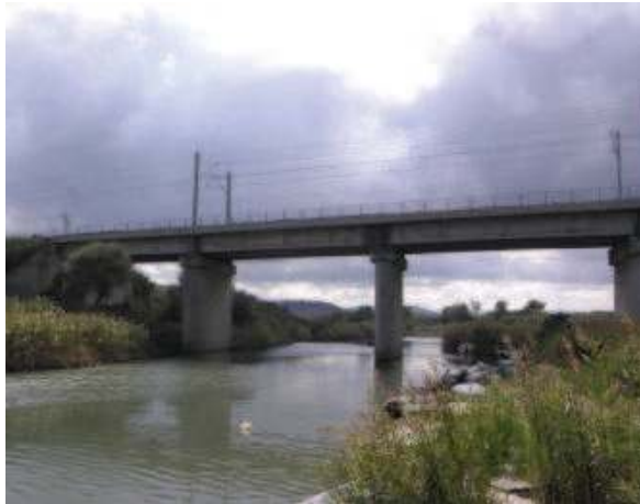
Fig. 1. Sinello railway bridge (Garibaldi et al., 2005).
