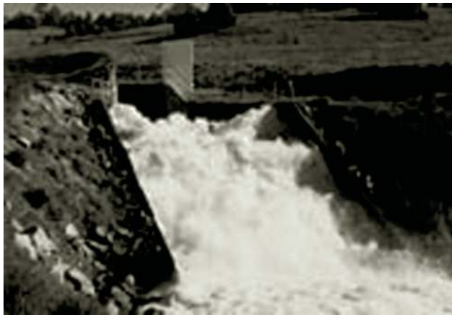
FIGURE 26.9 San Juan Chama Azotea tunnel outlet. (Courtesy of the U.S. Bureau of Reclamation.)
