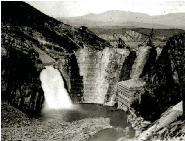
FIGURE 26.4 Roosevelt Dam under construction on the Salt River. (Courtesy of the Salt River Project.)
