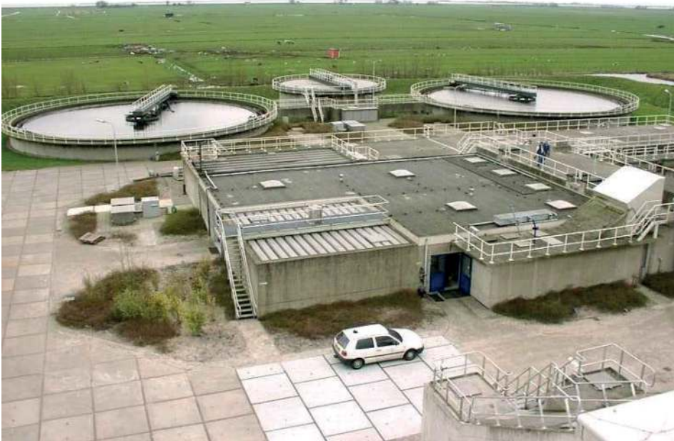
Figure 4.6 Images of WWTP Katwoude (Photo: Meijer S.C.F.).
