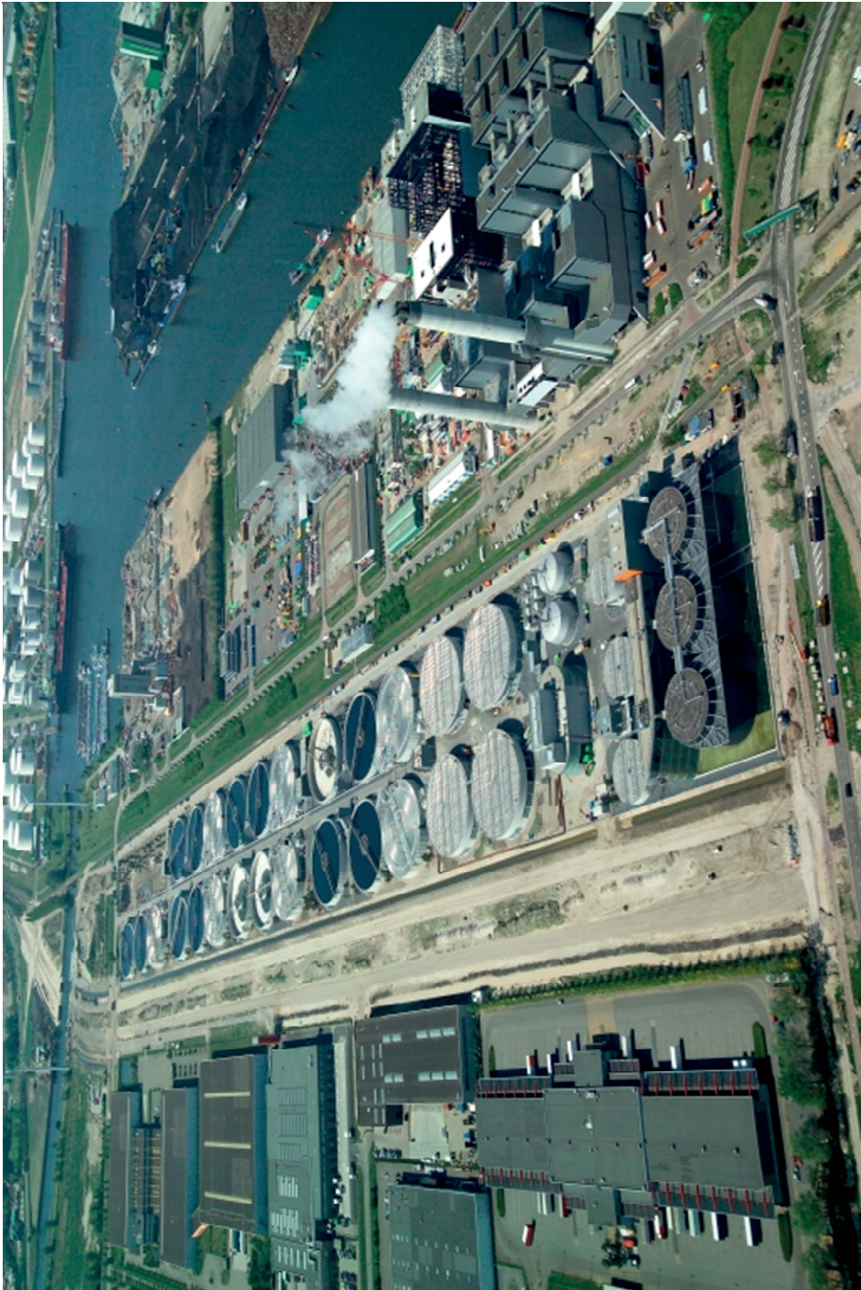
Figure 14.12 WWTP Amsterdam West (Photo: Waternet)
