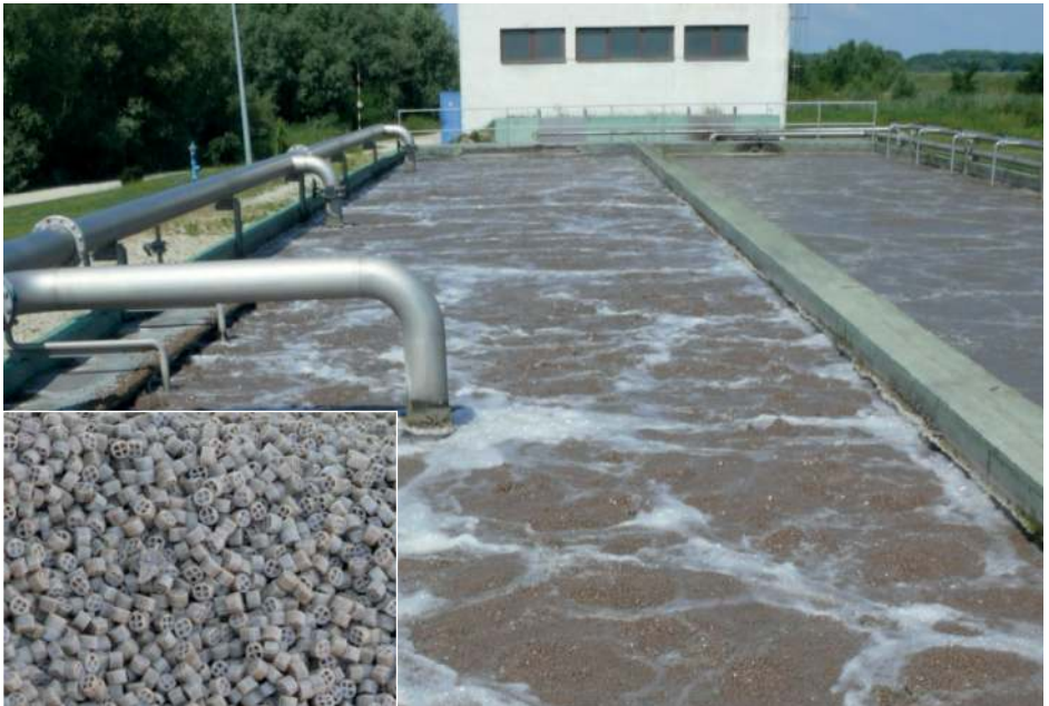
Figure 13.3 Biofilm carriers were introduced to increase efficiency of sewage treatment (photo: Brdjanovic D.).
