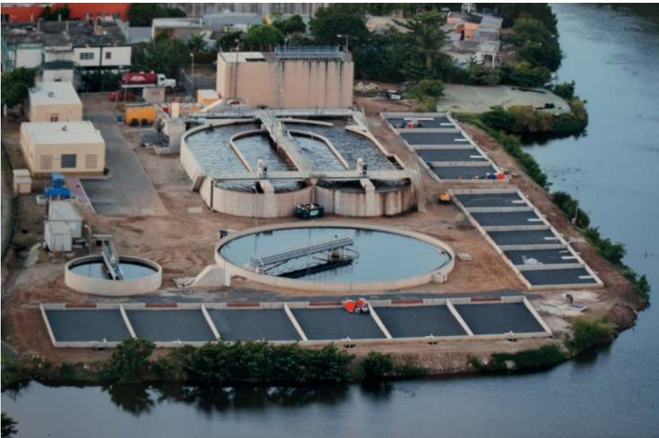
Figure 11.16 Aerial views of the old and new WWTP Illidge Rd. in operation (Photo: Buncamper C.).
