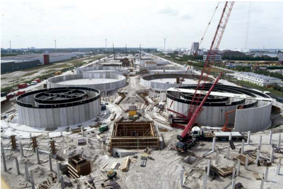
Figure 14.10 WWTP Amsterdam West during construction (Photo: Waternet)
