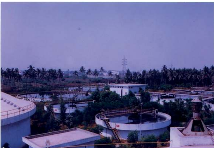
Figure 8.1 Wastewater treatment plant in Anjana.
