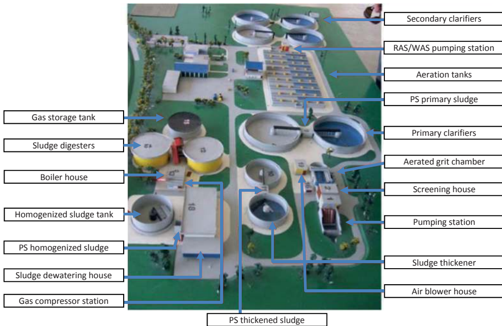
Figure 10.4 Model of WWTP in Sarajevo as built in 1984.
