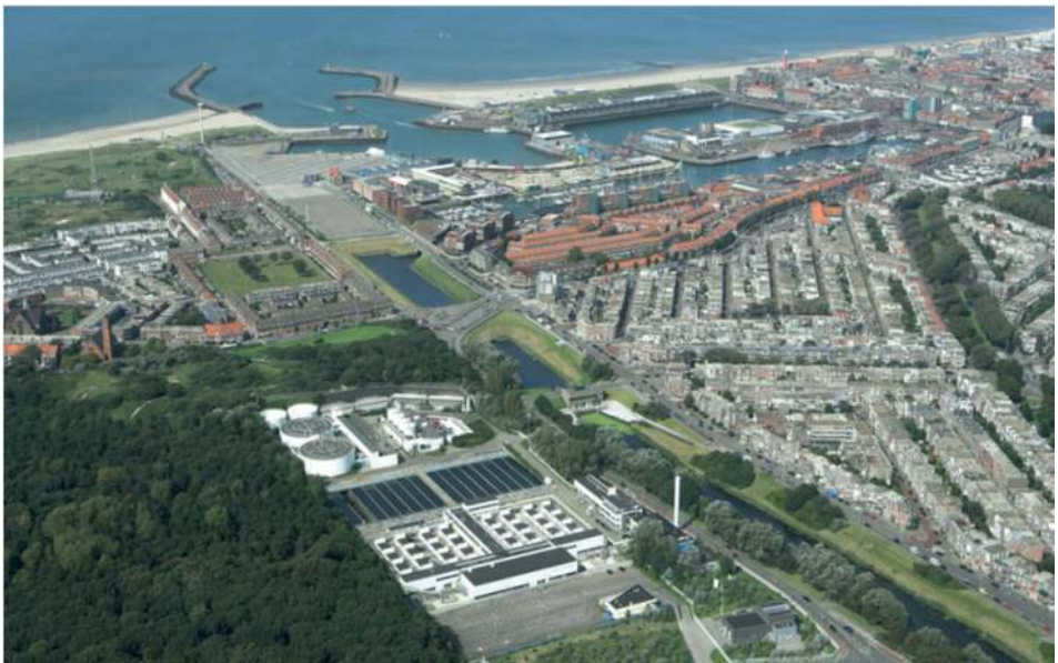
Figure 15.1 Aerial photograph of WWTP Houtrust in The Hague, The Netherlands. The Houtrust treatment plant is largely built underground. Below the parking lot are the primary setting tanks, selector, pre-denitrification, anaerobic and anoxic tanks. Eight activated sludge tanks are arranged in four lines and are covered (at the bottom of the photo). The thirty two rectangular secondary clarifier tanks are stacked in a double layer arrangement (middle section). The plant includes digestion and sludge processing (top section).
