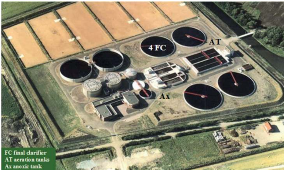
Figure 7.1 WWTP Walcheren, The Netherlands.
