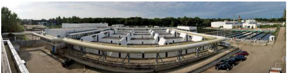
Figure 15.25 Panoramic view of WWTP Houtrust (Photo: Delfluent Services BV).
