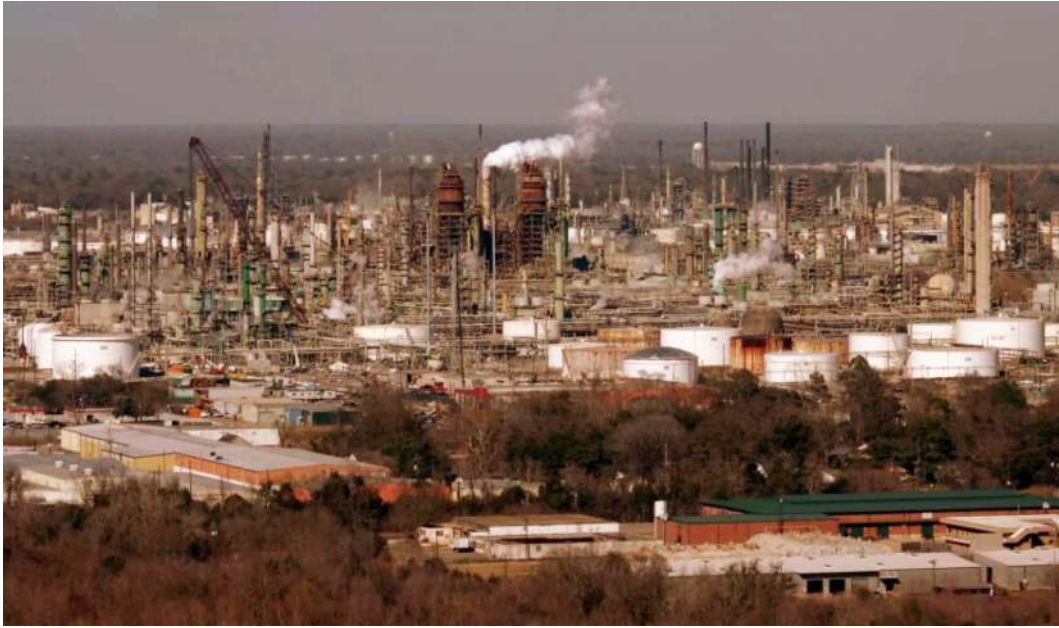
FIGURE 1. The ExxonMobil refinery in Baton Rouge on the Mississippi River, built in 1909, is one of the largest oil and gas processing facilities in the world. Louisiana has sixteen such refineries, none of them younger than fifty years old. Eight of them, incidentally, were found to be the worst water-polluting in the country—and five of them were among the top ten. A 2023 report by the nonprofit Environmental Integrity Project found that among the toxic polluters of nickel, selenium, nitrogen, ammonia, and “total dissolved liquids,” Louisiana’s aging refineries ranked at the top. ExxonMobil, for instance, ranked number 10 in the country for selenium discharges. There are two hundred industrial, petrochemical, and heavily polluting plants along the river corridor between Baton Rouge and New Orleans. Image available on Flickr through Creative Commons license by Jim Bowen.
