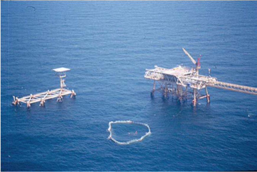
Fig. 13.5 Dunlop Tempest 4™ 18,000 m 3 cage system in 40 m of water at the platform site 54 km offshore on the central coast of Texas
