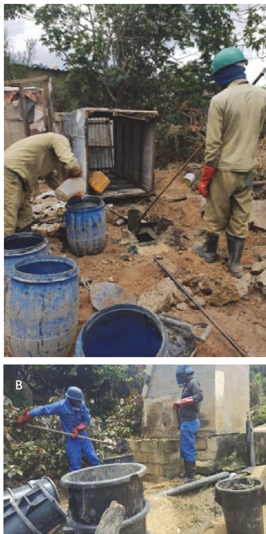
Figure 3.16 A) sampling during a manual emptying operation in Lusaka, Zambia, and B) Durban, South Africa (photos: Eawag).
