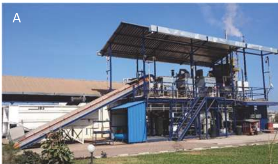
Figure 4.16 A) a contact dryer at the Omni-processor pilot plant at Niayes FSTP in Dakar, Senegal. In this plant, the sludge is incinerated leading to the generation of heat and electricity. B) part of the heat from combustion is recirculated in the process for the drying of the sludge with this contact dryer unit (photos: UKZN PRG).
