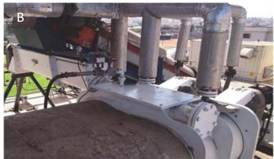
Figure 4.16 A) a contact dryer at the Omni-processor pilot plant at Niayes FSTP in Dakar, Senegal. In this plant, the sludge is incinerated leading to the generation of heat and electricity. B) part of the heat from combustion is recirculated in the process for the drying of the sludge with this contact dryer unit (photos: UKZN PRG).
