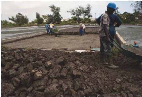
Figure 2.10 Removal of semi-solid to solid dewatered sludge from drying beds at Camberene treatment plant in Dakar, Senegal (photo: Eawag).
