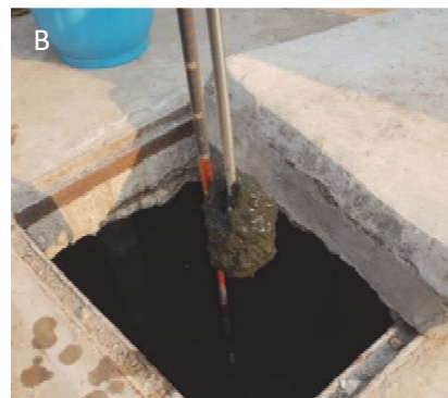
Figure 3.3 A) taking a core sample from a septic tank in Lusaka, Zambia, and B) the sampling device becomes clogged if the sludge is too thick. This example shows the collection from a 10-year old septic tank that had never been emptied. The tank was leaking, and so the supernatant leached out into the soil, resulting in a very thick sludge accumulation (photos: Eawag).
