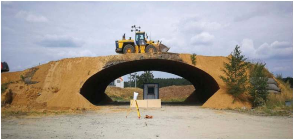
Figure 1. View of the loaded structure.
