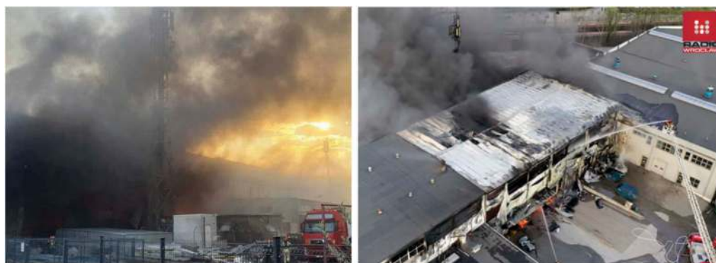
Figure 2. Fire in the warehouse adjacent to the tower (source: left – Gazeta Wrocławska; right – Radio Wrocław).
