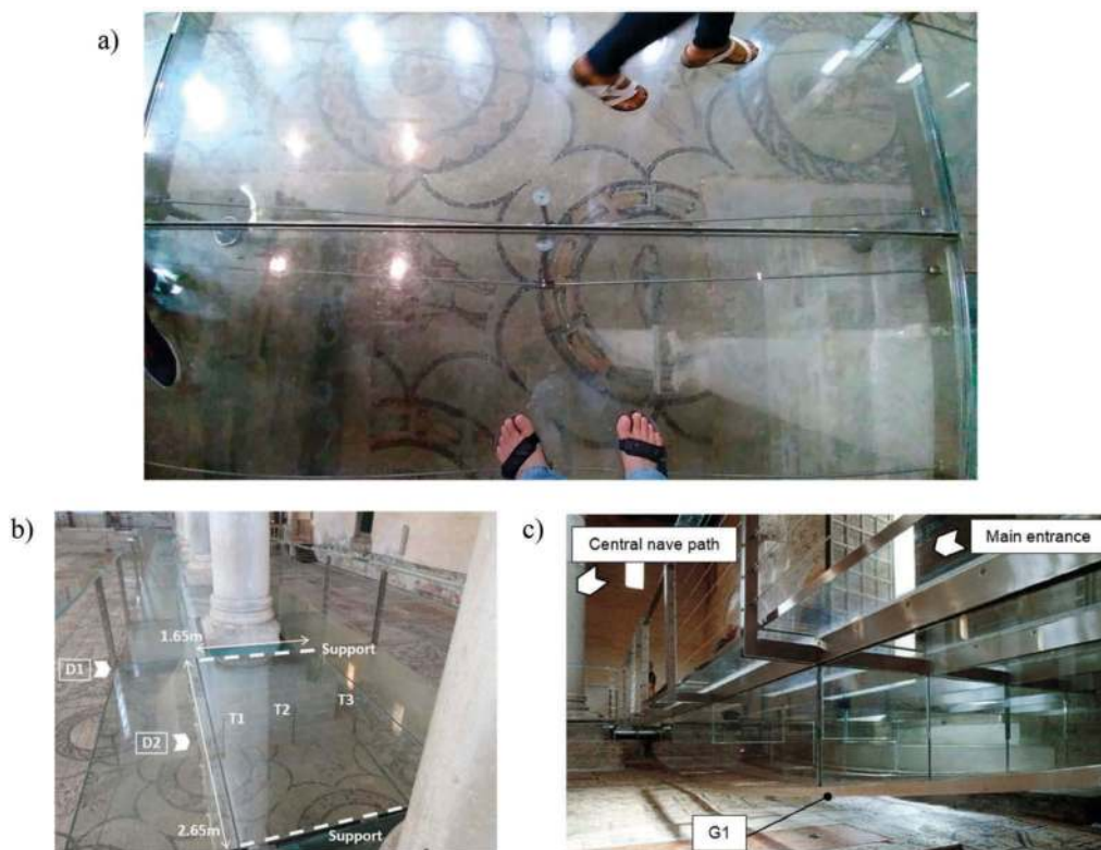
Figure 7. Vibration analysis of an existing in-service glass walkway: a) visual inspection and b) - c) details of the structural system. Figures reproduced from (Bedon & Fasan, 2019) under the terms and conditions of the Creative Commons Attribution (CC BY) license).
