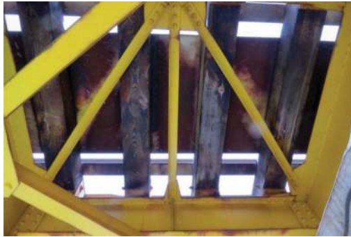
Figure 2. View of the bottom of the structure – elements, from which samples were collected.
