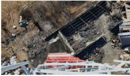
Figure 4. The adjacent area subjected to fire – the warehouse (top view).
