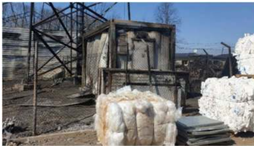
Figure 5. The telecom shelter destroyed during the incident.
