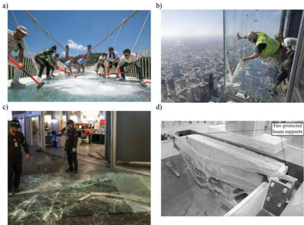
Figure 3. Structural glass applications in buildings: a) bridge; b) balcony; c) envelope collapse due to blast and d) laminated glass beam in fire testing (reproduced from (Bedon, 2017) under the terms and conditions of the Creative Commons Attribution (CC BY) license).
