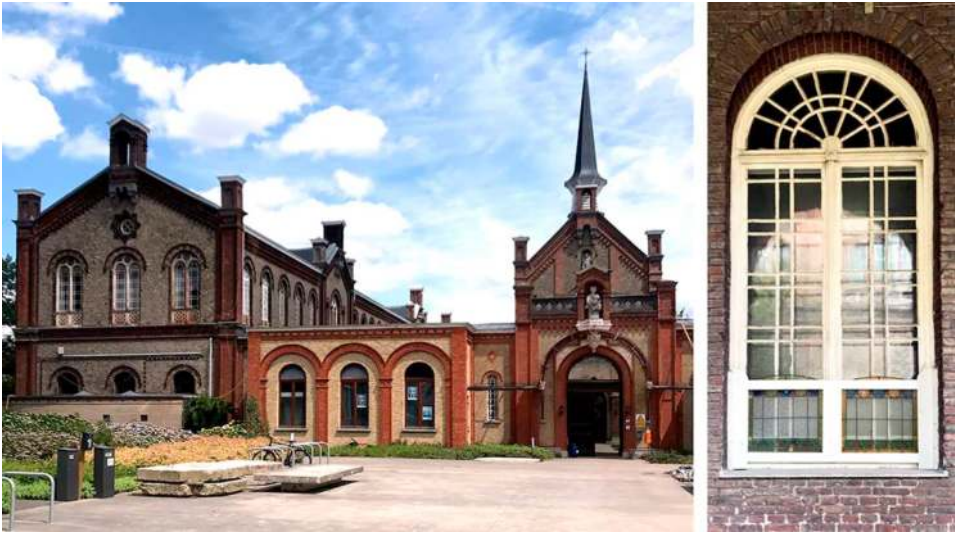
Image 1.2 The former Guislain asylum in Ghent (1857), photo of the main entrance and window detail.
