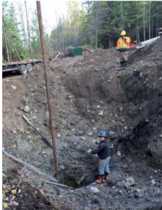
Figure 9. Views of site E with wood crib within the shoreline forest of Smith's Bay. Figure is from November 1, 2016, and shows the excavation in progress with the discovery of a barrel at ~5 m below grade but still 4 m above the well box [21].
