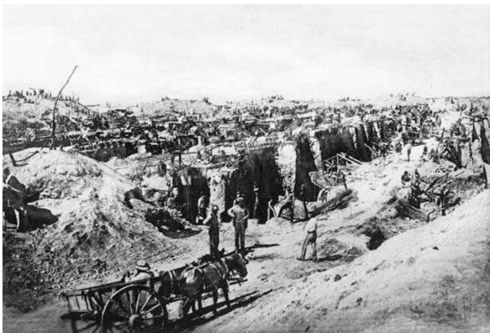
Only linking roadways remained
