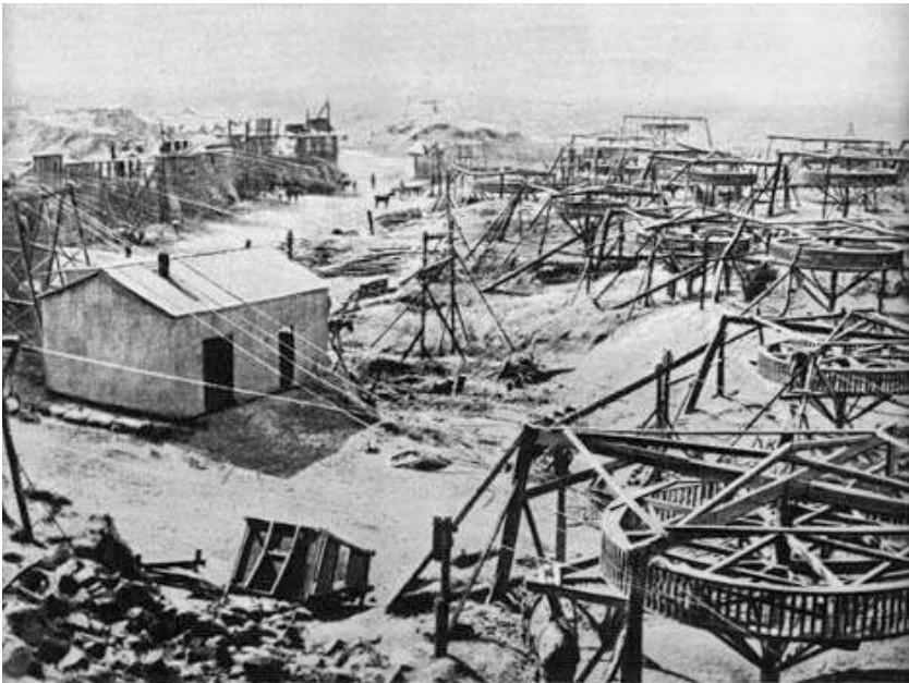
Horse-driven winches at the Kimberley mine
