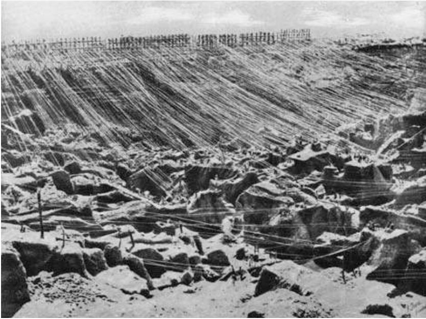
Cables for the mining bins
