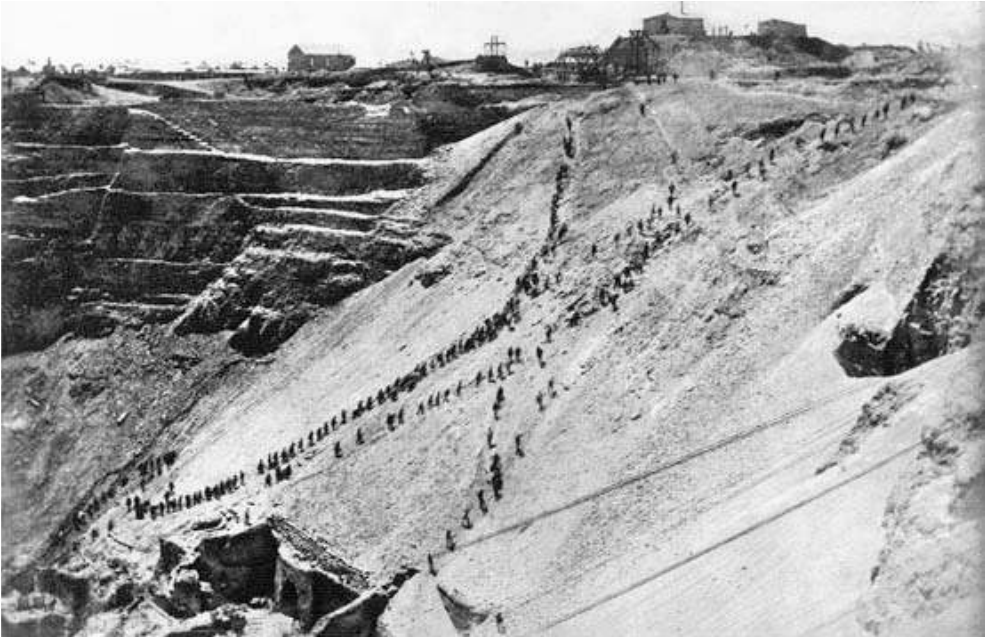
End of the working day
