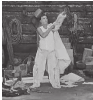
Figure 0.3 Donning the Asbestos Suit
