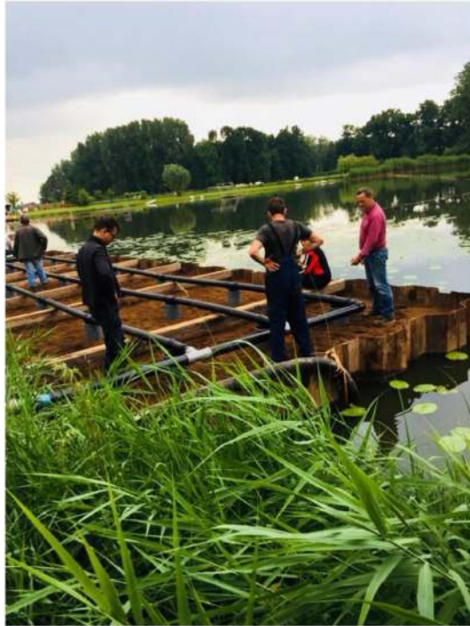
Figure 12.5 Application of iron-rich drinking water sludge as a means to minimise eutrophication in lakes (photo credits: Olaf van der Kolk, Aquaminerals).
