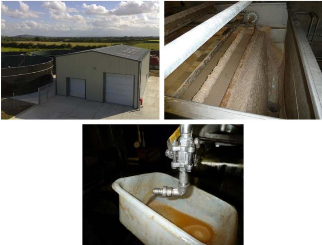
Figure 12.4 The case study plant overview (left top), the dissolved air flotation with 'fat' flotation sludge (right top) and the recovered fat (bottom).
