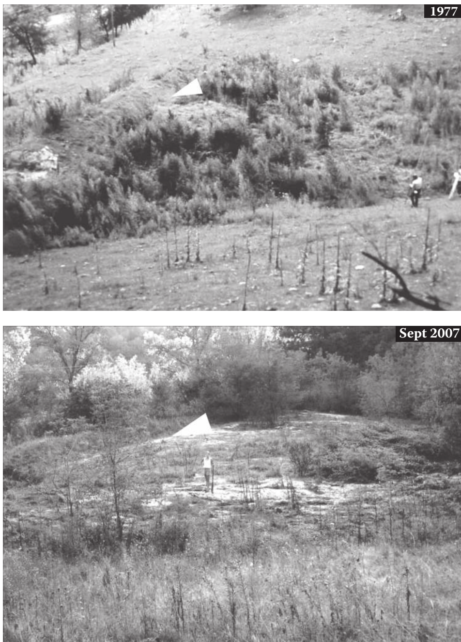
Figure 8.10 Upper Mitchell debris basin, built in 1941 to protect WI Hwy 56 from gully debris, 4 mi (7 km) SE of Genoa ( P = 10\text{--}12 in. or 30 cm, Sec 36, T13 N R6W). Top: Surveying the basin, 1977. Basin filled in 4 years (1941–1945). Dam to left, sediment basin outlined by dark vegetation, Hwy 56 to top left. Arrow marks edge of fill against dam. Bottom, September 2007. Light material is 1–5 in. (2.5–7.5 cm) of sediment delivered by August 2007 storm. Note that level of fill by dam is hardly higher than in 1977.
