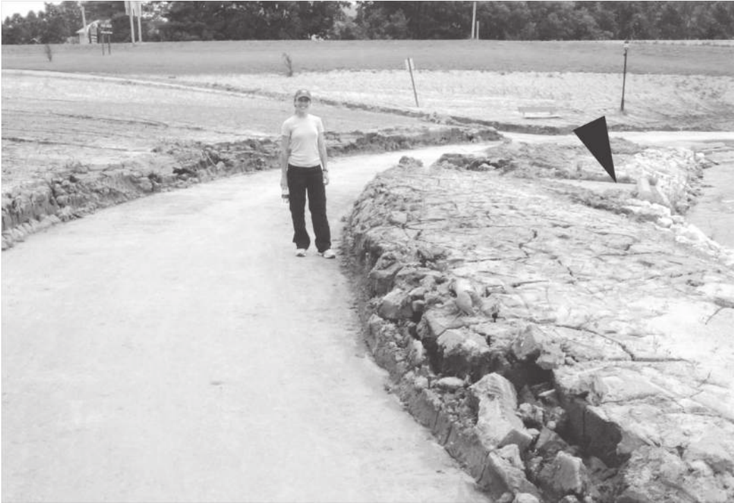
Figure 6.4 Aggrading “new” floodplain in Coon Valley Village Park. Floodplains were cut down to facilitate handicapped access ramps (arrow) to Coon Creek (seen on far right). Subsequently, the stream has attempted to rebuild its floodplains to the height dictated by the present flood regime, that height being about 6 ft (2 m). The elevation of the lowered floodplain is shown by the paved walk on which the person stands, and the recent deposits are up to 2 ft (60 cm) thick. However, the formerly retreating high banks have been stabilized with rock so that the previously expanding floodway is now stable and is decreasing in size. Photo made July 2008.
