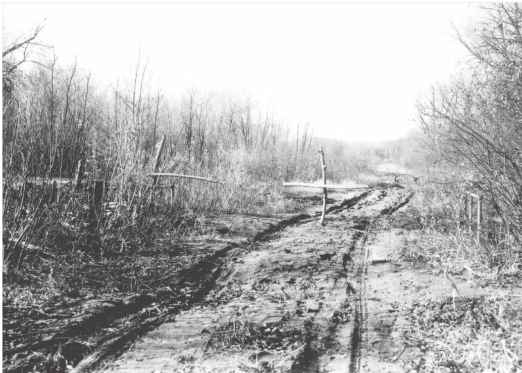
Figure 7.22 Minnesota State Aid Highway 9 on the south side of the Whitewater River, 11/6/37. Bridge in right foreground was covered by 18 in. (45 cm) of sediment by June 1938. This road, the lifeline for people on the south side of the river, was becoming impassable by the late 1930s. By 1989, it was underwater, impassable even on foot. (Photo credit Soil Conservation Service [SCS].)
