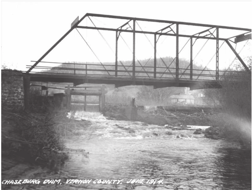
Figure 7.4 Bridge over Coon Creek on Mill Street in Chaseburg just below auxiliary dam (seen in background), looking southwest (upstream), June 1914. Note rock shoals below dam. The sills of the bridge were about 13 ft (4 m) above the water. For locational reference, note Lutheran church in background. (Continued)
