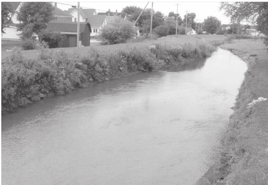
Figure 7.17 Arcadia, WI. Turton Creek at an old mill site, looking downstream towards the Trempeleau River, 2011. The stream flows along the north side of the town. Note that the water surface of the creek at normal flow is presently almost as high as the land on the other side of the flood dike. The dike to the left is about 4 ft (1.2 m) high. The fact that most of the houses in town had a basement suggests that the original water level was at least 10 ft (3 m) lower. Even the level of the millpond here would have been considerably lower than the present level of the stream. Otherwise, it would have flooded the areas to either side and would have raised local groundwater levels. The higher present stream levels, including the Trempeleau River, just 2 mi (3 km) downstream from this site, have caused groundwater to rise and flood basements in the town.
