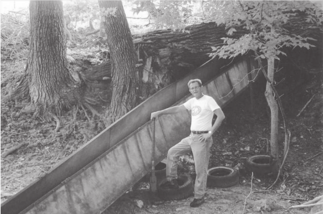
Figure 3.5 Early private erosion control. Sheet metal flume used to convey water around the head of gullies, Proksch Coulee gully, Vernon Co., WI (see Chapter 4). (Photo credit: Nadine Kleinhenz.)
