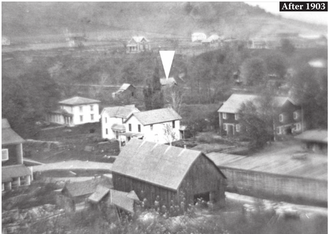
Figure 7.3 (Continued) Chaseburg, refer to Figure 7.1 and 7.2. View to the northeast. Martiny house west of Main Street marked with arrow. Dark building with white trim to far left is the mill. The white Italianate building to the right of, and beyond, the mill is the village hotel. In the background is the site of the “new” town. Photo date unknown but after 1903. (Continued)
