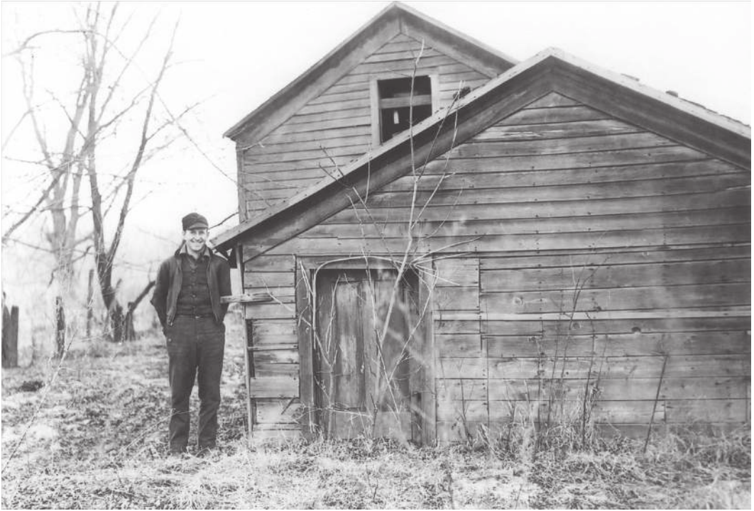
Figure 7.10 A partially buried house in Beaver, 11/28/39. See H. Johnson (1976, pp. 212-213) for another example).
