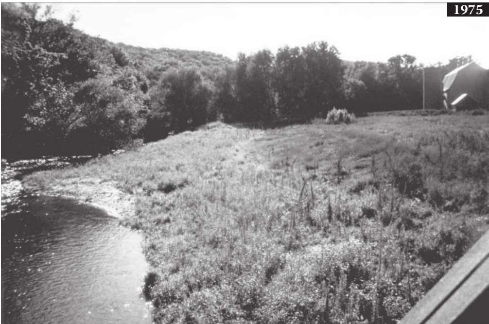
Figure 8.11 North Fork of Whitewater River 1 mi (1.6 km) west of Elba, looking upstream from bridge as seen in Figure 3.12; note barn for reference. Top: 1940. Note disturbed condition of channel. Bottom: 1975, condition was stable, and this has continued to the present. (Continued)
