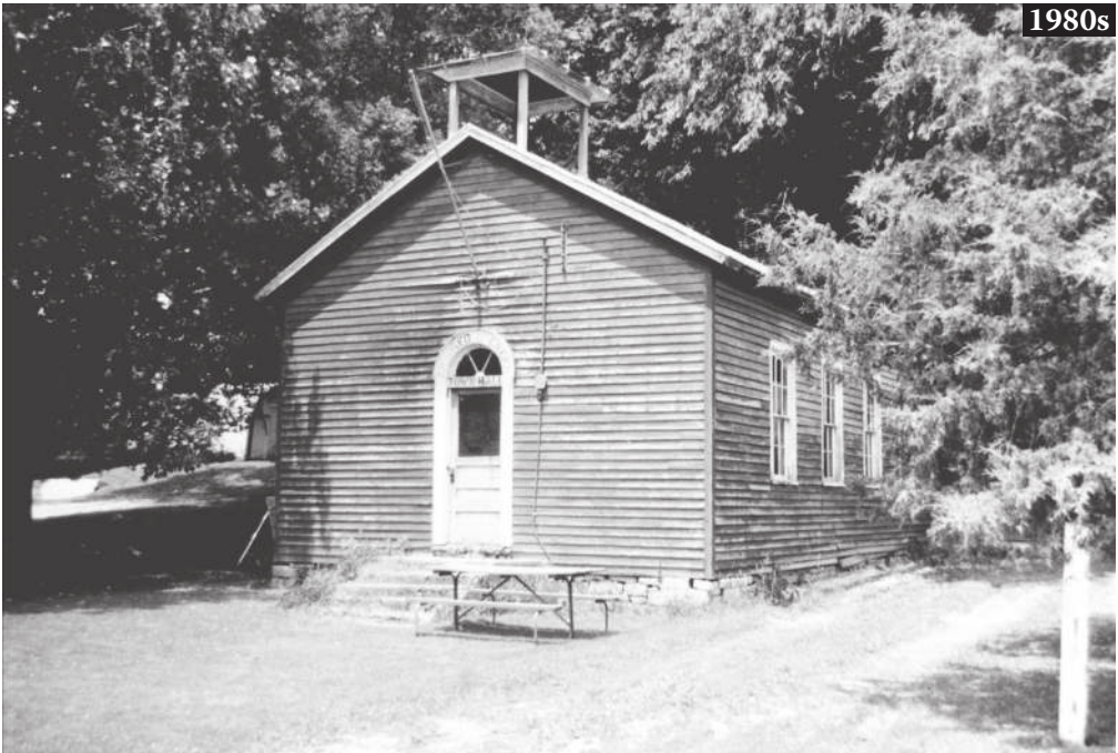
Figure 6.5 Freeburg, Crooked Creek, Houston Co., MN. Crooked Creek Township Hall. Top: Turn of century, photo made from road. Viewer's eyes are at a level about 4 ft (1.2 m) below the bottom of wooden siding on the building. Bottom: Again standing on the road, 1980s. Viewer's eyes are level with bottom of first board below windows. This suggests that road is now about 8 ft (2.5 m) higher.
