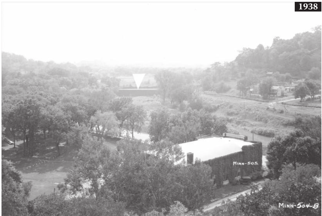
Figure 5.13 Lanesboro Lake, Lanesboro, MN, on the upper Root River. C. 1890: large expanse of water. 1938: completely filled with sediment. Arrow marks top of dam in both photos. (Photo credit Soil Conservation Service [SCS].)
