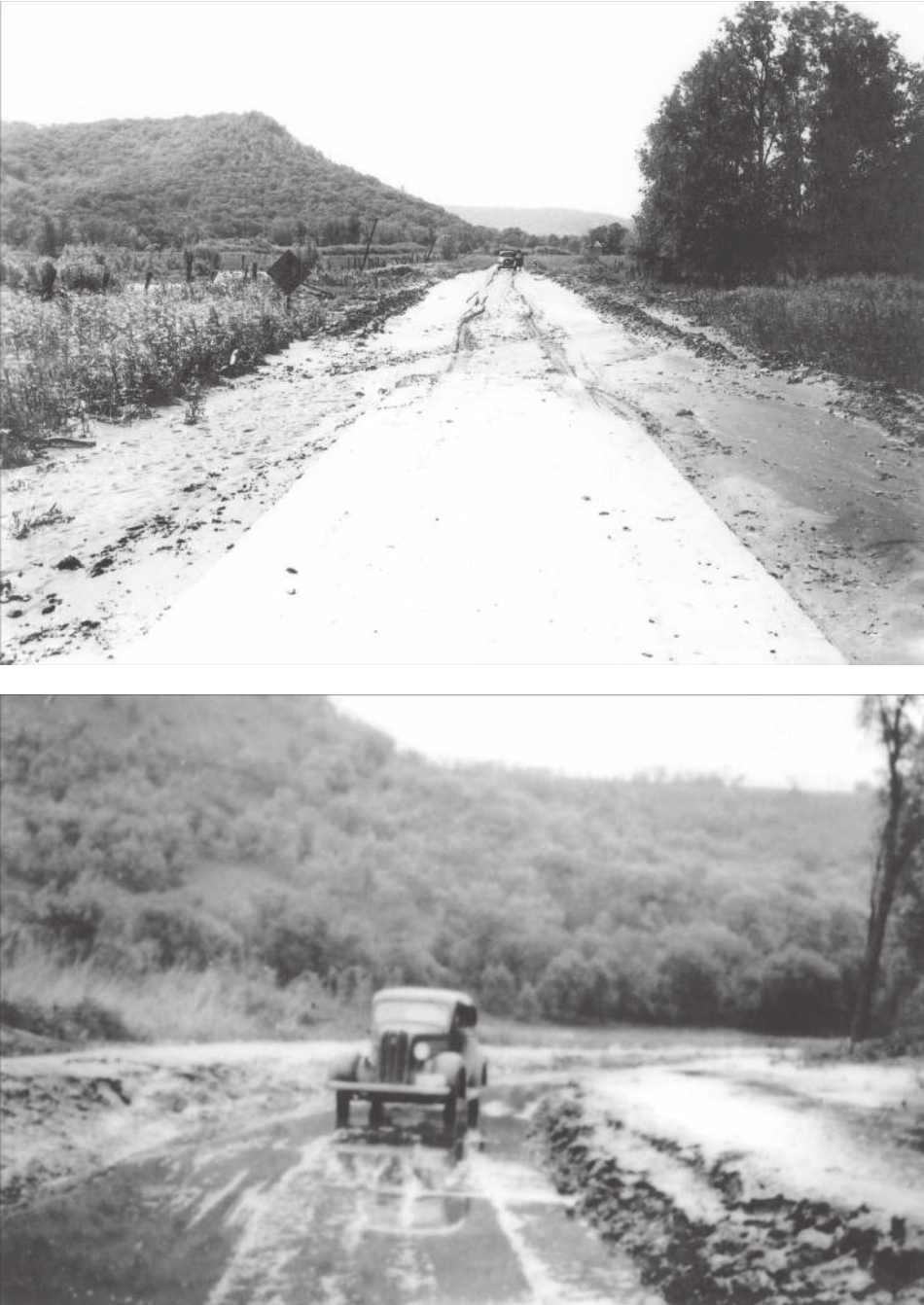
Figure 7.21 Minnesota State Highway 74 along the north and west side of Whitewater River on the floodplain. In an attempt to escape the increasing flooding and sediment accretion, it was built in 1918 on a 6 ft (2 m) high embankment with a narrow concrete roadway. By the late 1930s, the floodplain had aggraded to the level of the road or even above it. Top, 6/2/38 near Beaver. Bottom: Reach of Highway 74, probably near Beaver. The floodplain had aggraded above the highway, which had to be cleared.
