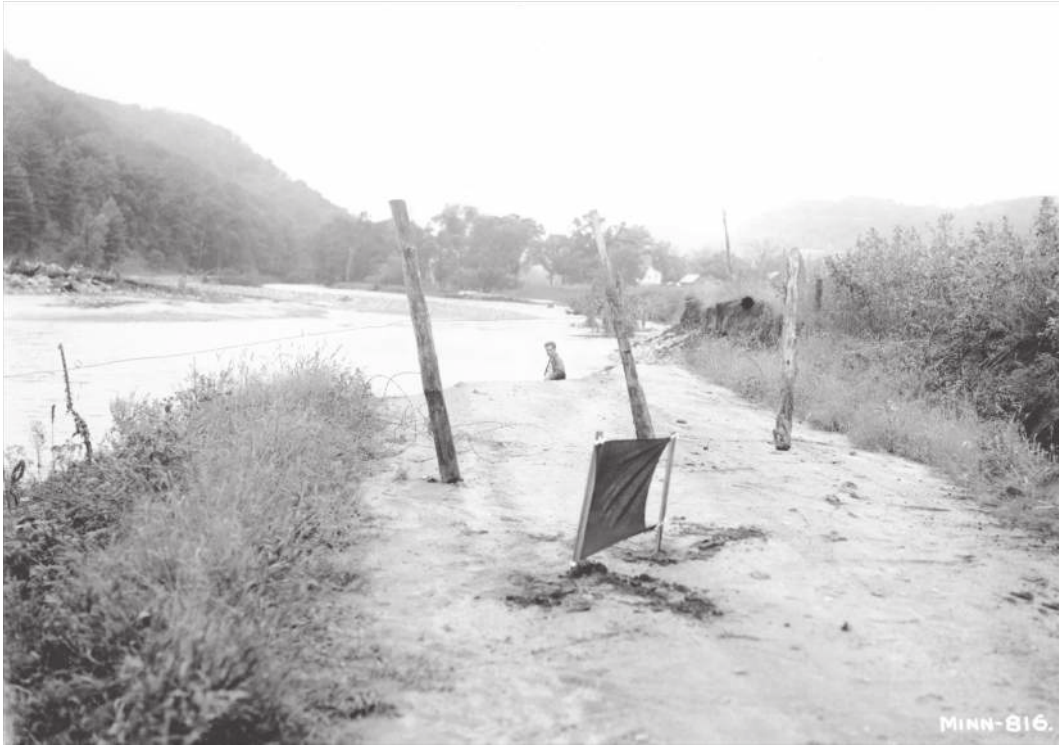
Figure 5.6 Fairwater, road from Elba to Fairwater about 1 mi east of Fairwater, 9/38, looking west. Several hundred feet of roadway eroded away.
