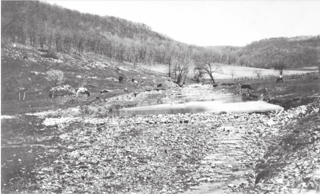
Figure 5.11 Oium Mill dam site, Timber Coulee, Coon Creek basin (N1/2, Sec8, T14N, R4W, Vernon County, WI), looking upstream from bridge on Lars Hill Road, 1919. Note typical “gravel road” appearance of stream and the almost lunar, bare quality of the heavily grazed landscape behind it. The expendable rock dam, rebuilt after every flood, diverted water into a race (to the right, not visible) that led to a reservoir excavated into a terrace downstream. This was above most floods thus saving it from destruction. The mill was about ¼ mi (400 m) downstream at the edge of the terrace (Files of Wisconsin Railroad Commission).
