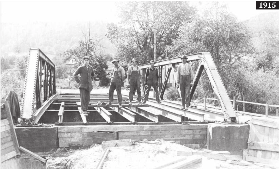
Figure 7.7 Early harbingers of a dark future for lower Chaseburg. Looking northwest at the cheese factory on south side of town, early 1900s. Floodplain of tributary from south in foreground with buried fence posts by road (now County Road K). Chaseburg cheese factory to left. For reference, Lutheran cemetery in right background. Bottom, raising the Main Street (now County Road K) bridge over the millpond on south side of village, 1915 presumably, to place it above floods. This channel is now completely occluded.
