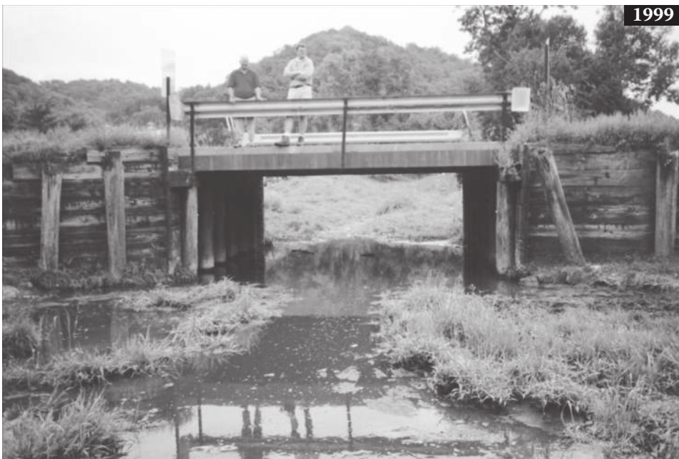
Figure 4.6 The Zink farm. Standing on fan looking east (upstream) at bridge on County Road O. Top: 1975. Wingwalls of buried earlier bridge are still visible. An excavation 5 ft (1.5 m) deep here in 1975 and 1976 did not reach the base of the wingwalls nor did it fill with water, indicating the lack of permanent flow and significant underflow at that time. Bottom: 1999. The wingwalls have been buried in the aggrading fan. Most notable to observe is the permanent streamflow, which began in 1988. For scale, the person to the right is 77 in. (193 cm) tall.
