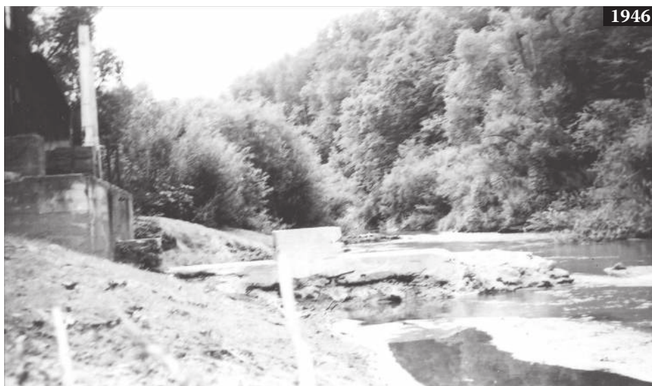
Figure 7.5 (Continued) The main dam at Chaseburg looking upstream; refer to Figure 7.2. 1946. Dam has been demolished and is rapidly being buried. Note rectangular concrete pier on dam to hold flash boards, probably a delaying tactic to keep the mill going a few more months. (Continued).
