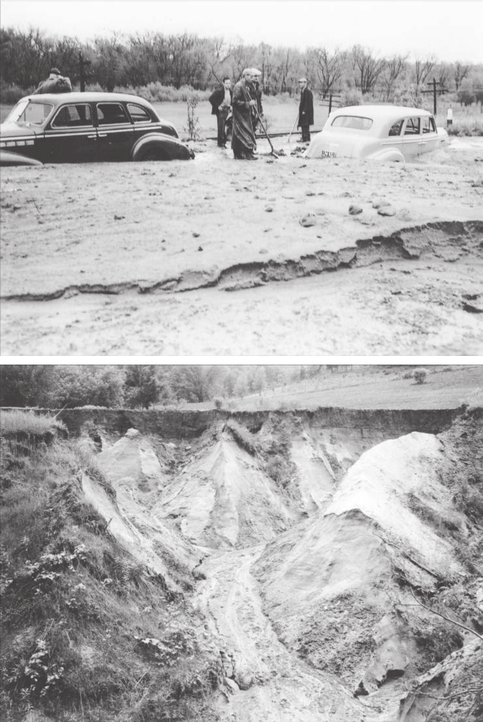
Figure 4.8 Top: cars halted and partially buried by sand fan on US Highway 61 about 2.5 mi (4 km) north of Weaver, Wabasha Co., MN, 6/7/40. The fan covered 0.2 acre (0.08 ha), was 7 ft (2.1 m) thick at the apex, and contained 4.6 acre-feet (5,700 m 3 ). Bottom: The gully that created the fan, 6/9/40. Note the almost vertical walls. (Photo credit Soil Conservation Service [SCS].)
