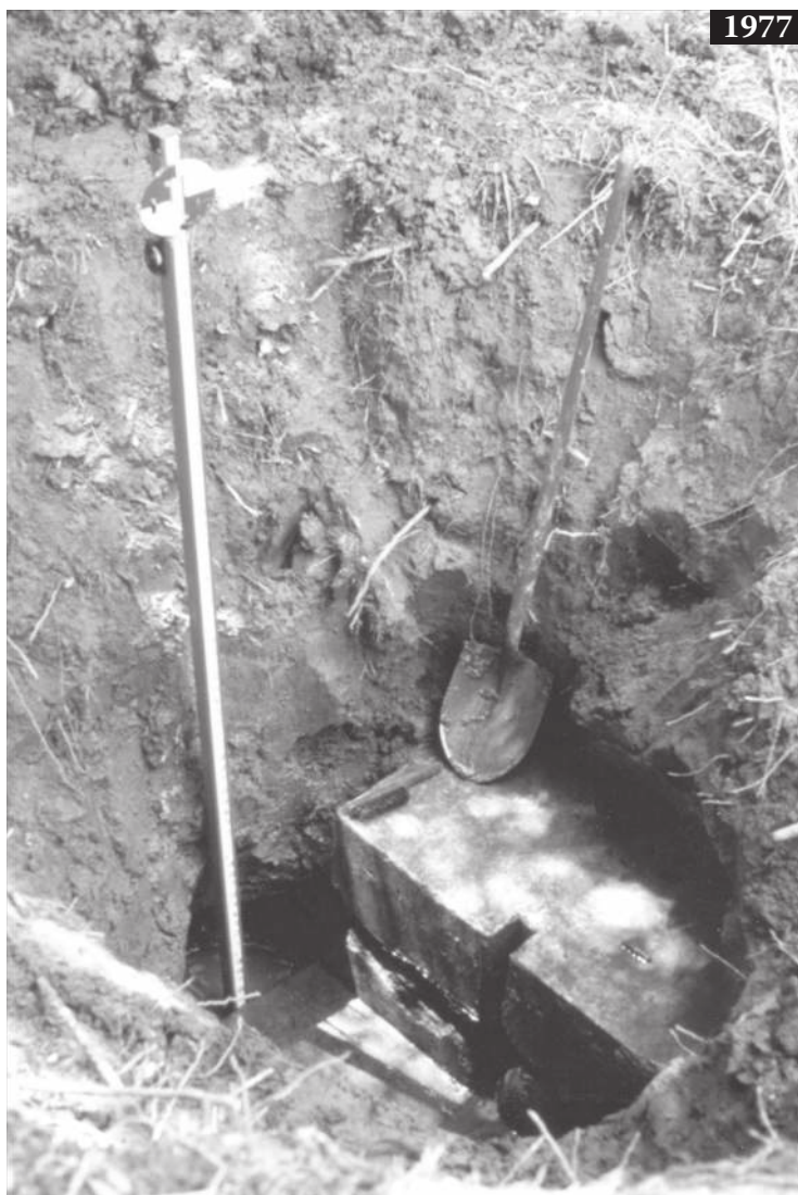
Figure 7.5 (Continued) 1977. Rectangular pier to hold flashboards (seen in the 1946 photo), excavated 1977. An elevation placed on the dam in 1932 tied into earlier surveys by the WI Dam Commission and allowed reconstruction of village elevations back to 1914 (Figure 7.2).
