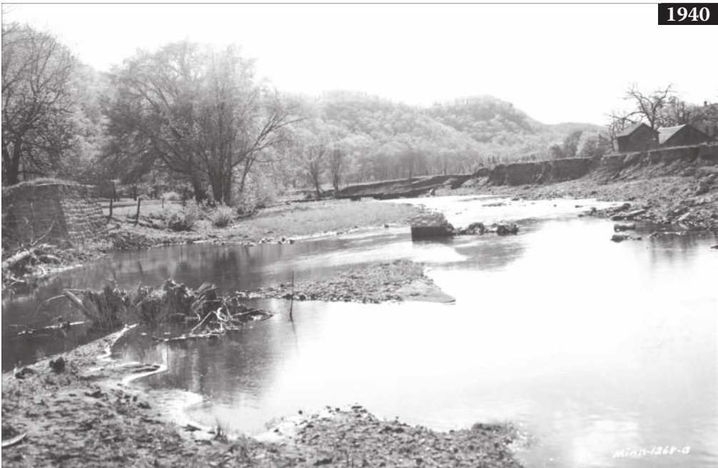
Figure 5.5 Fairwater, bridge crossing visible in 5.1 and 5.2 looking upstream. c. 1905: the structure is probably slightly later than the one visible in 5.1 and 5.2 but is at the same crossing. Note stability of stream and banks. 1940: stream widened by about three times here so that right pier is near the center of the widened stream. The left pier is still visible (2006) in the village, but the recovering (narrowing) stream has buried the right pier in the new bank.
