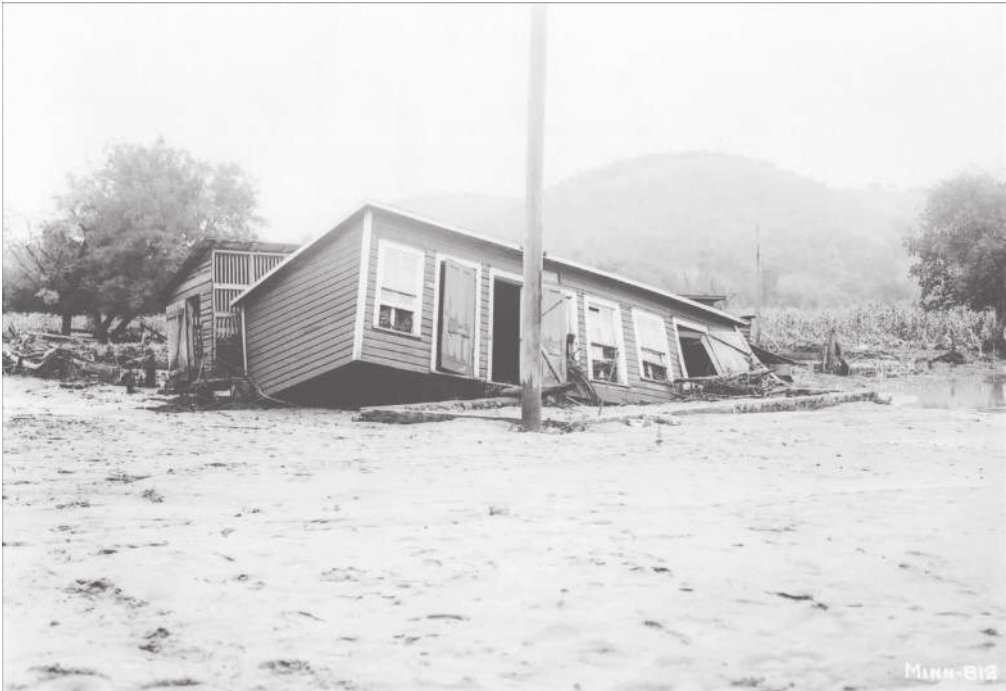
Figure 6.1 Nick Siebenaler's house just upstream from Elba, MN, on a terrace above the Whitewater River. Flood 9/8/38. Top: Floodwater was up halfway on screen door. The men are pumping out the basement. Bottom: Siebenaler's chicken house was moved off the foundation by the flood. Note sediment deposits in foreground. (Photo credit Soil Conservation Service [SCS].)
