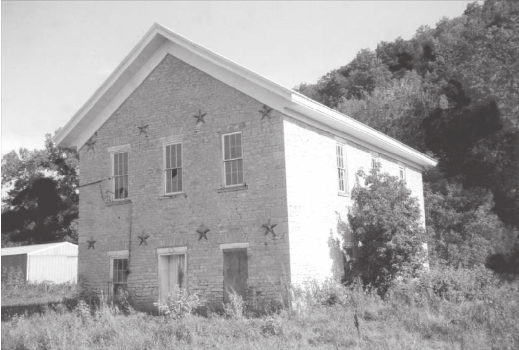
Figure 7.15 Village Creek. The schoolhouse, built in 1860, is the only old building left. Although in a higher part of the village, it has been buried 4 ft (1.2 m) so that downstairs windows are at ground level. (Photo credit: Nadine Kleinhenz, 2006.)
