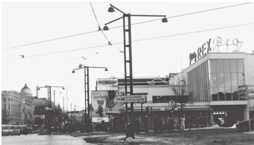
Half of the centre's buildings are older architecture. Strong feelings about these buildings have made authorities protect them. The Glass Palace was restored in the late 1990's by the City of Helsinki and now serves as a centre for modern media. It houses a movie theatre (Bio Rex), television broadcast studios, internet library and media café. Photo: Jorma Kivistö.
