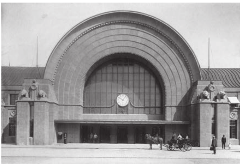
The Railway Station designed by Eliel Saarinen and Herman Gesellius. The beautiful station building was blown up during the retreat of the Russians in 1941. Photo: South Karelia Museum, Lappeenranta.
