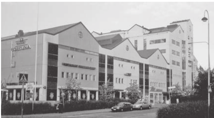
A small supermarket, post office, office for social security and few small shops make everyday life easier and also offer opportunities for inhabitants to meet other people socially. Photo: Jorma Kivistö.
