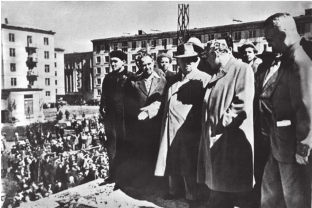
Nikita Khrushchev (third from the right, in the center of the front row) at an experimental construction site on Shchemilovka Street in Leningrad, 23 May 1957. Photograph by V. Kapustin. Central State Archive of Documentary Films, Photographs, and Sound Recordings of St. Petersburg, Br 18377. Reprinted with permission of the TSGAKFFD SPb.
