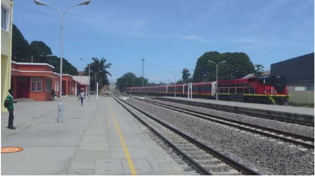
Figure 11.1 The CFB train pulls into Catumbela station.
