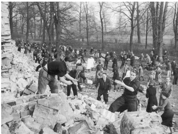
Figure 12.1 Clearing up the rubble: making space for the new Tierpark, 1955. Bundesarchiv Berlin 183-29610-002, Zentrabild Quasch. 26.3.1955.
