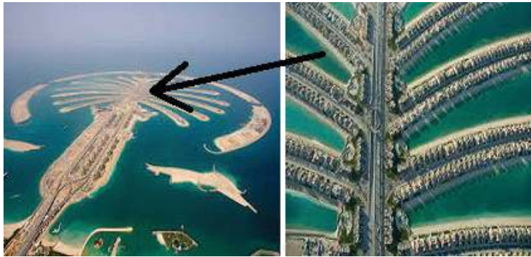
Figure 19. Residential complex in Palm Jumeirah, Dubai.
